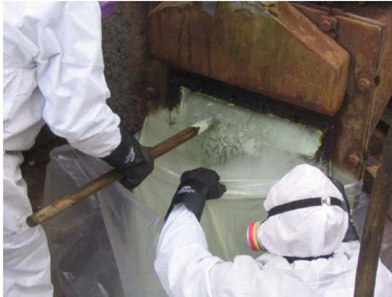
PHOTOGRAPH 17 FIRST PHOTOGRAPH: EMPLOYEE REMOVING DIOXIN AND HCB CONTAMINATED ANONDE DUST FROM GRIZZLY BOX SECOND PHOTOGRAPH: EVIDENCE OF SMOKING INSIDE GRIZZLY BOX CONTAINMENT PIT PHOTOGRAPHS TAKEN JULY 26 2006
