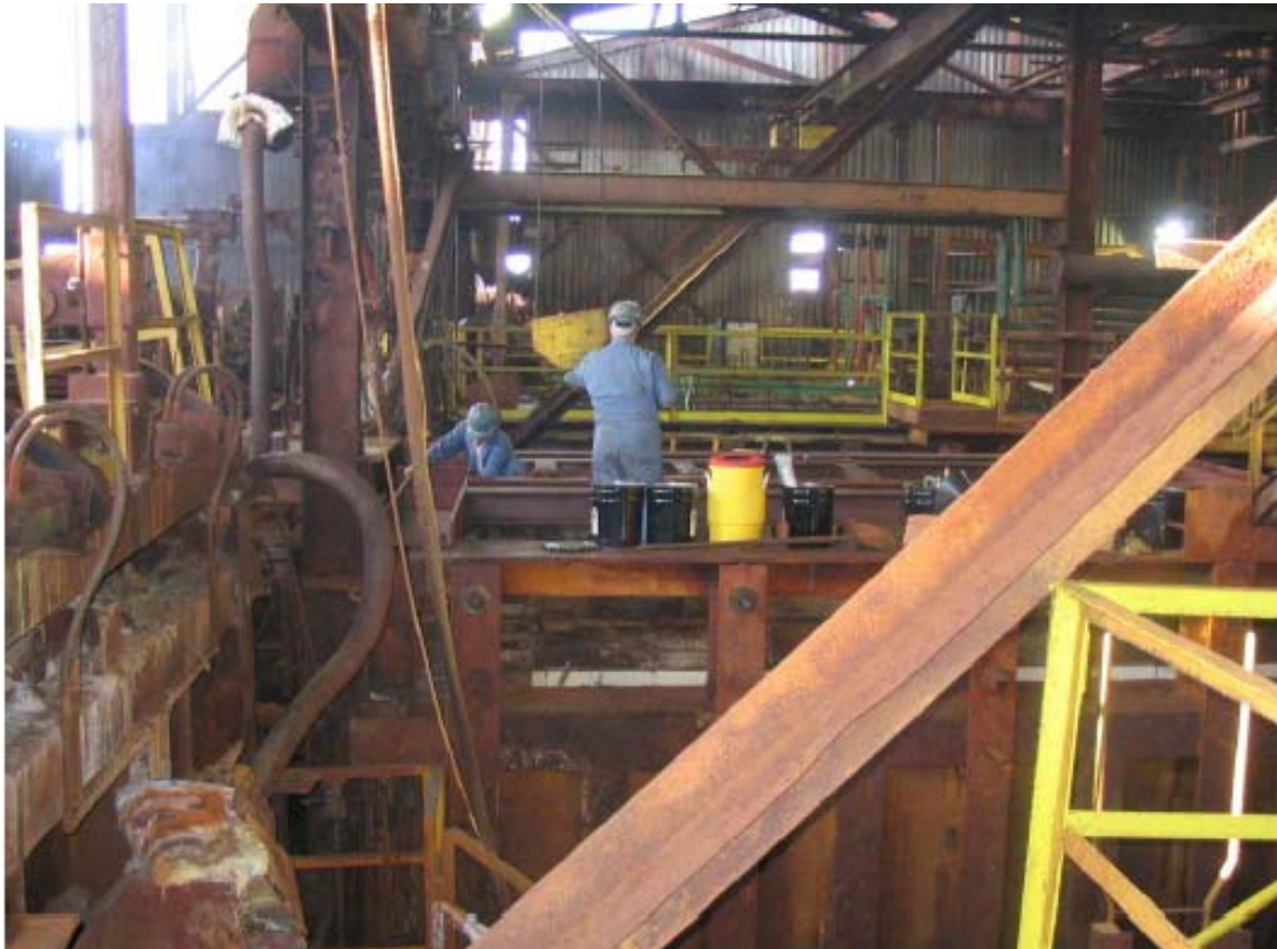
PHOTOGRAPH 3 EMPLOYEES WELDING I-BEAMS-6 TH FLOOR REACTOR BUILDING WORKING WITHOUT RESPIRATORS PHOTOGRAPHS TAKEN JULY 26 2006
