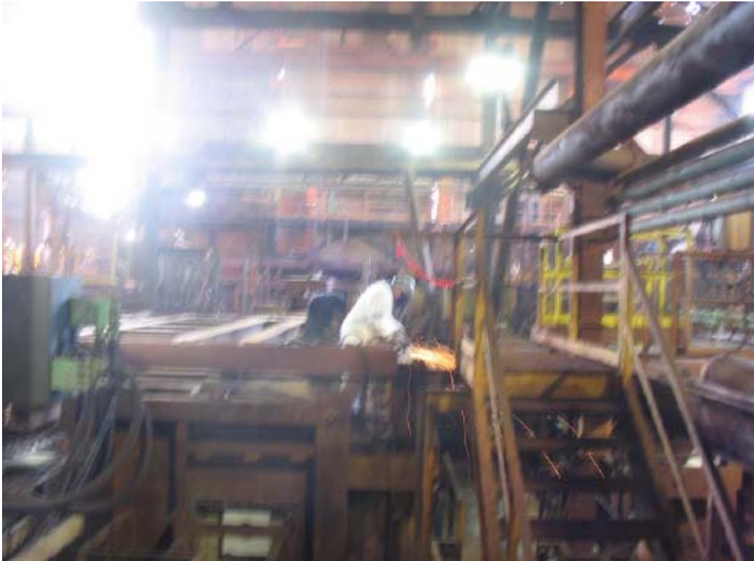
PHOTOGRAPH 6 WORKER WELDING I-BEAMS-6 TH FLOOR REACTOR BUILDING WORKING WITHOUT RESPIRATORS GENERATING WELDING FUMES PHOTOGRAPH TAKEN JULY 26 2006
