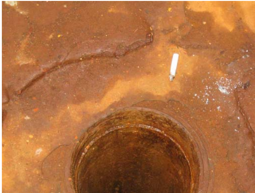
PHOTOGRAPH 14 EVIDENCE OF SMOKING AND DRINKING INSIDE THE MELT REACTOR BUILDING PHOTOGRAPH TAKEN JULY 26 2006
