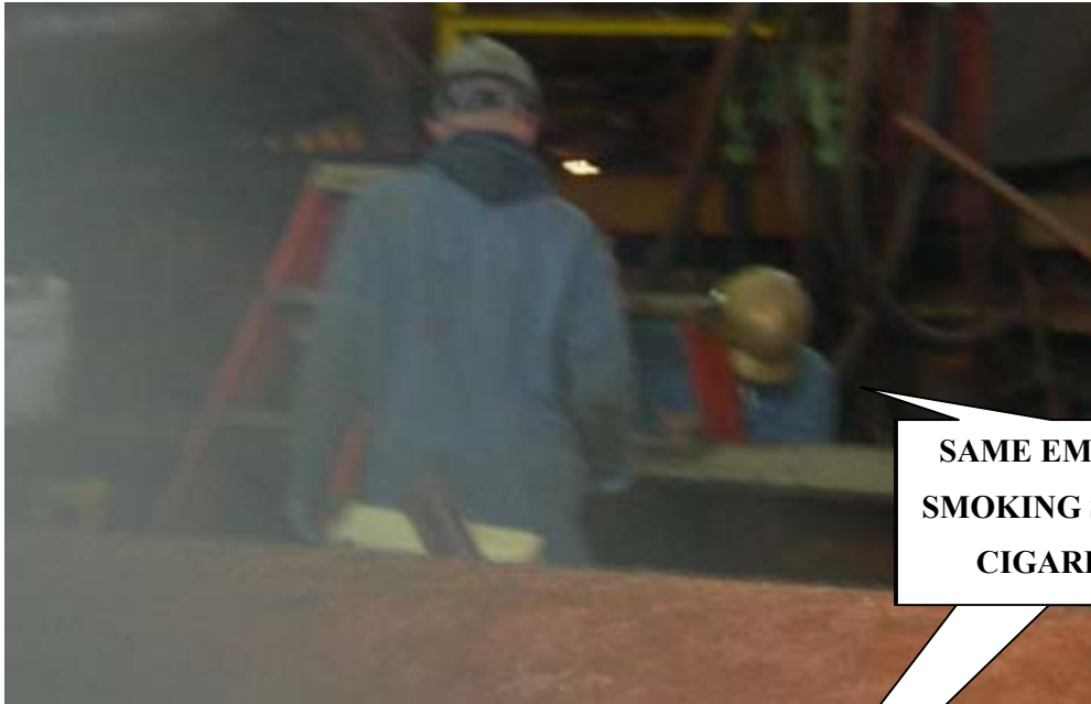
PHOTOGRAPH 15 REACTOR CELL REBUILD WORKERS-6 TH FLOOR REACTOR BUILDING NO RESPIRATORS AND SMOKING WHILE REBUILDING REACTOR CELL PHOTOGRAPH TAKEN SEPTEMBER 20 2006
