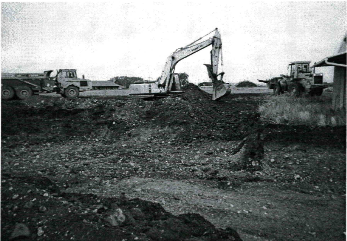
Excavation of Pit areas South of Peeler building.
