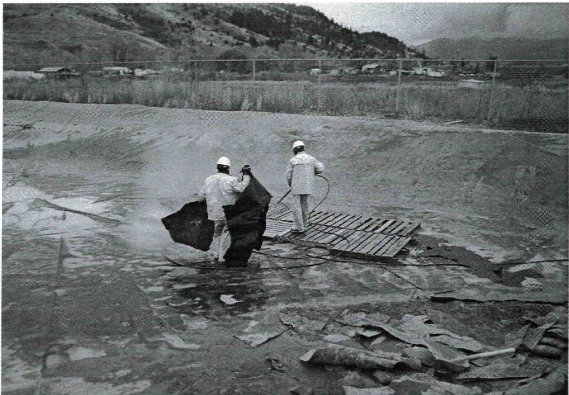
Original liner washing area in the bottom of the Retention Pond.
