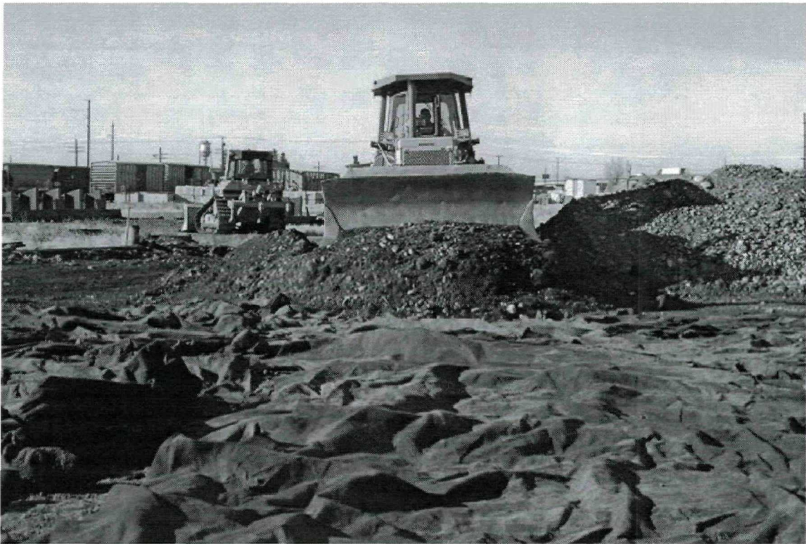
Dozer pushing clean soil cover over geo-textile above backfilled treated LTU soils.
