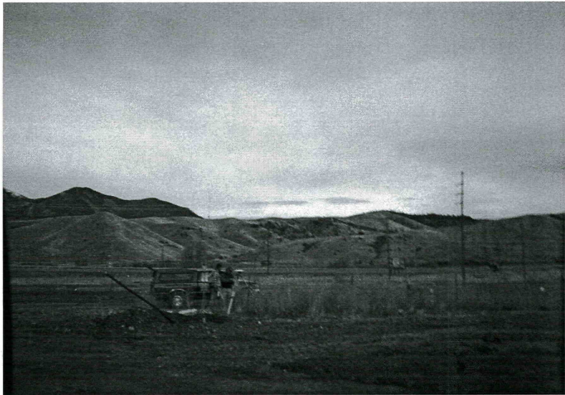
Surveying surface of treated LTU soil placement South of PP-Injection Gallery.
