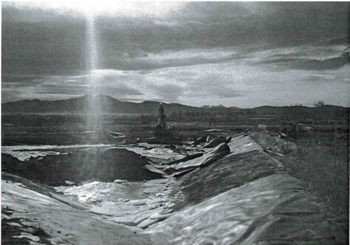
Removing liner from Retention pond.
