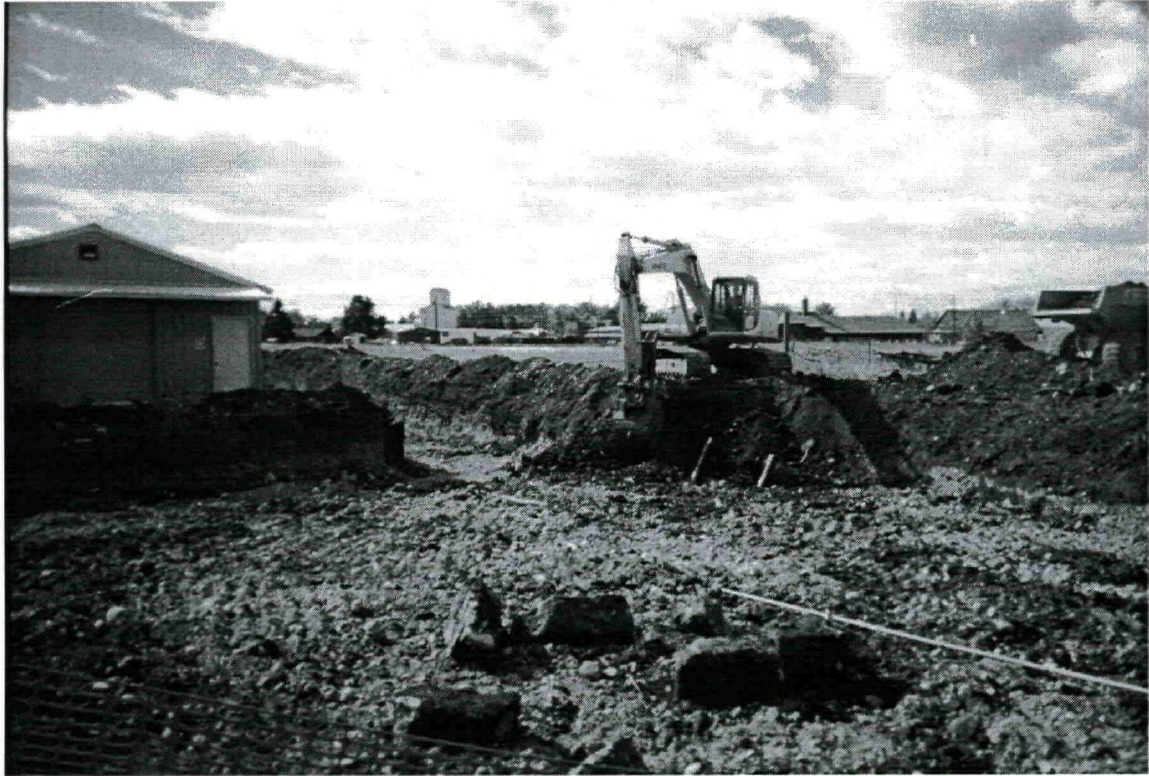
Excavation of Pit areas around peeler building.
