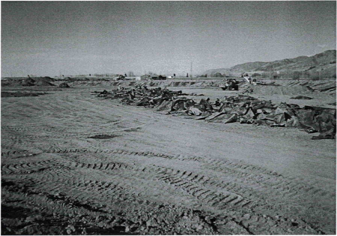
Stockpile LTU liner prior to pressure washing.
