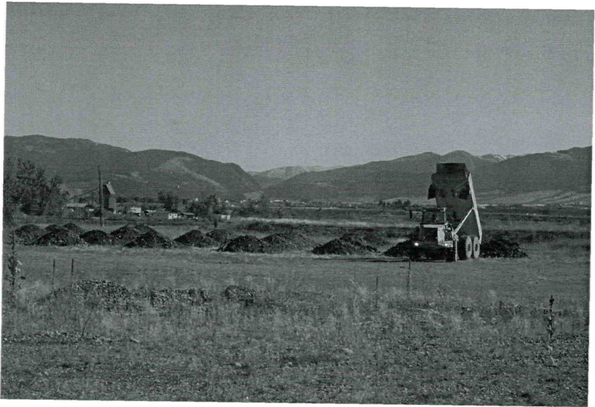
Clean fill excavated from Pits 5 & 6, and placed in low area East of PP-Injection gallery.
