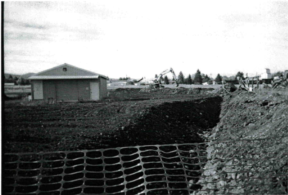
Treated LTU soils backfilled into Pits 5 & 6 (Day 7).
