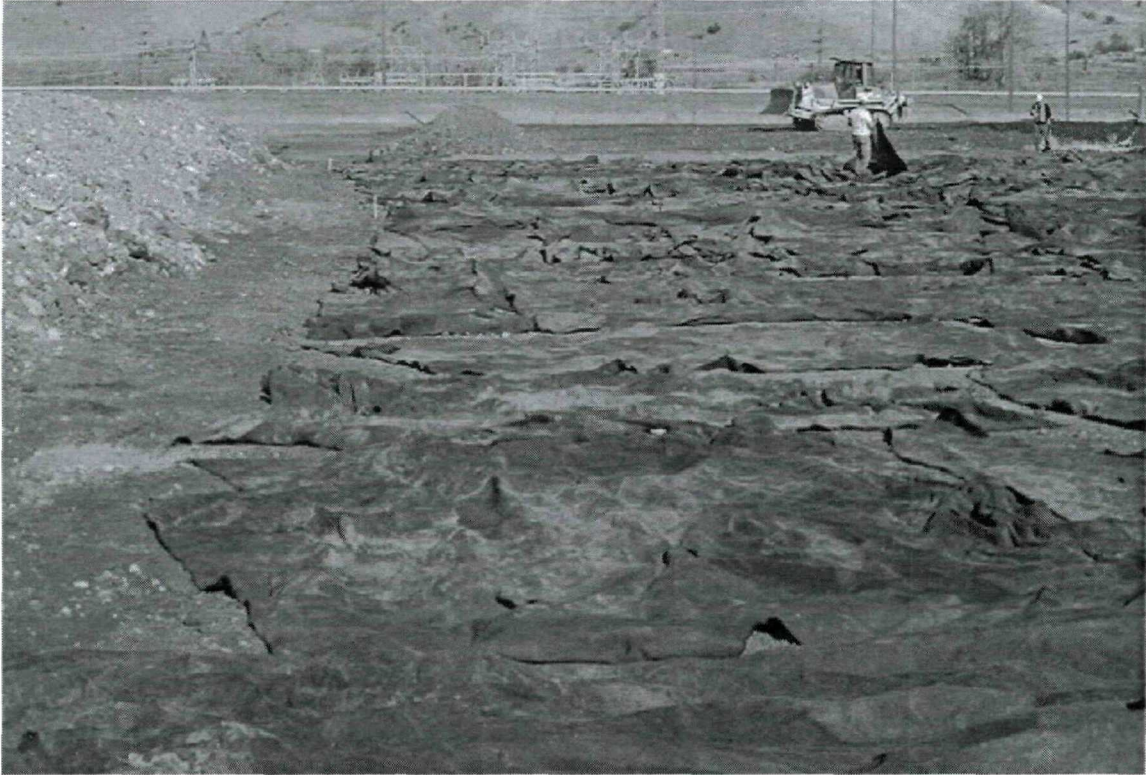
Placement of Geo-textile fabric on treated LTU soils in Pit areas.
