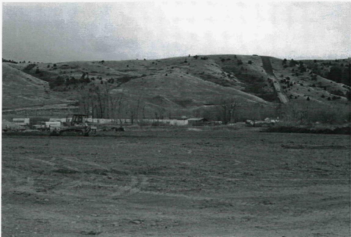
Finish grade of LTU area.
