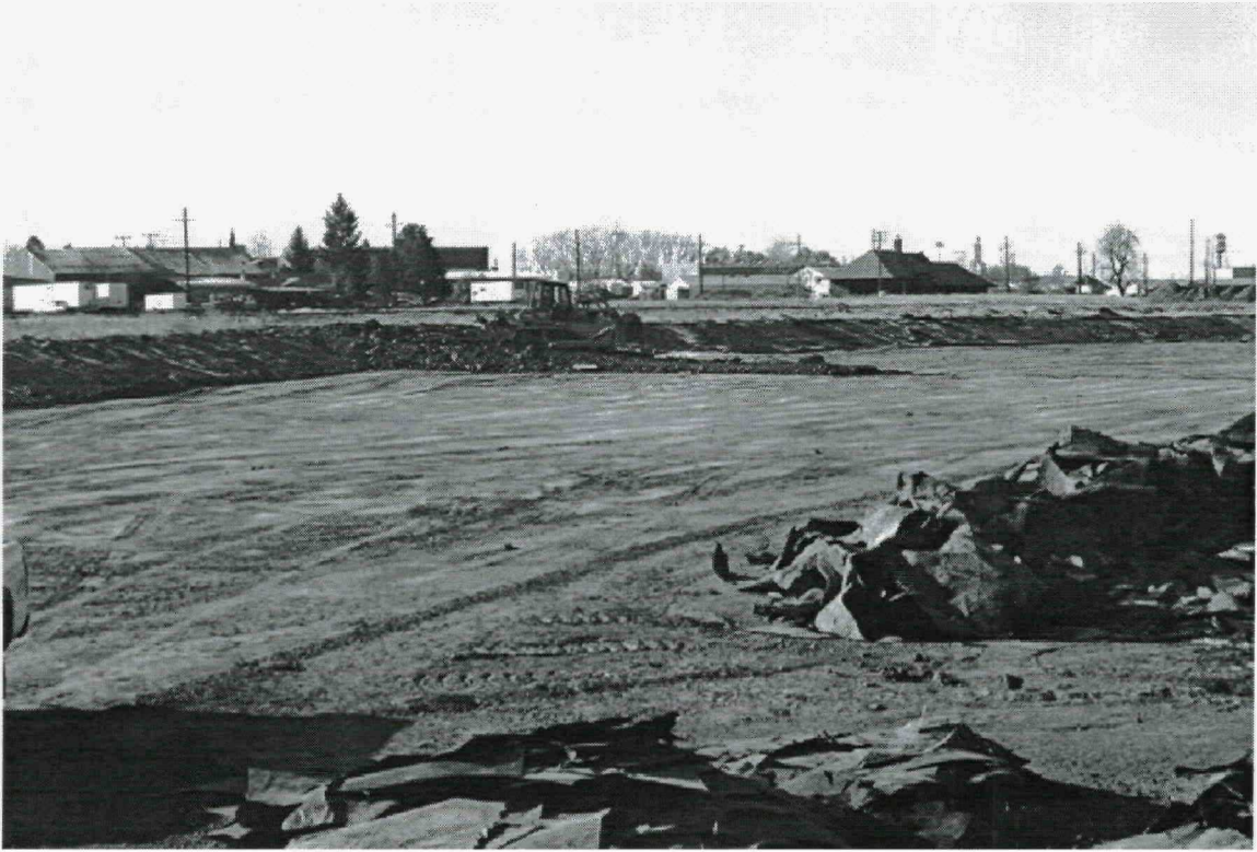
Dozer pushing in LTU berms upon completion of soil removal.
