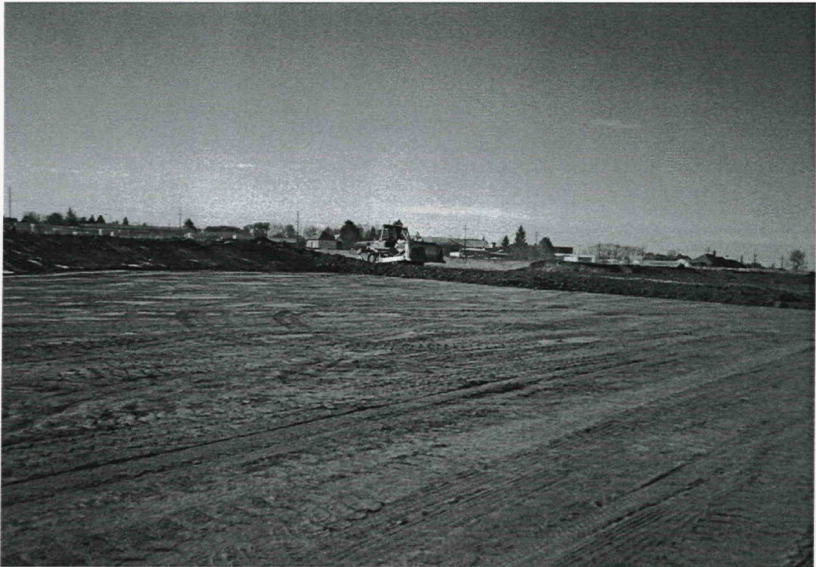
Dozer pushing in berms of LTU for final grade.
