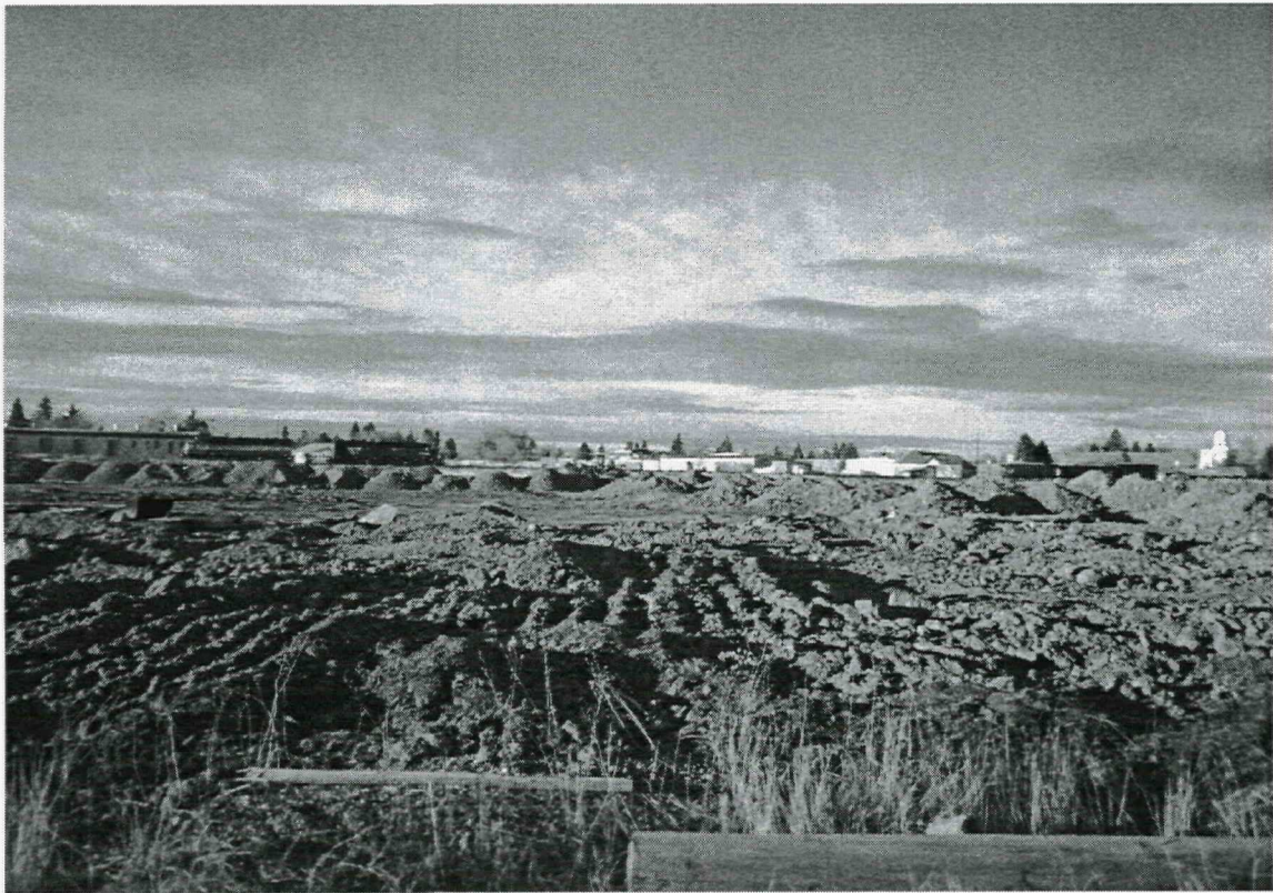
Clean soils staged on LTU area for final grade.
