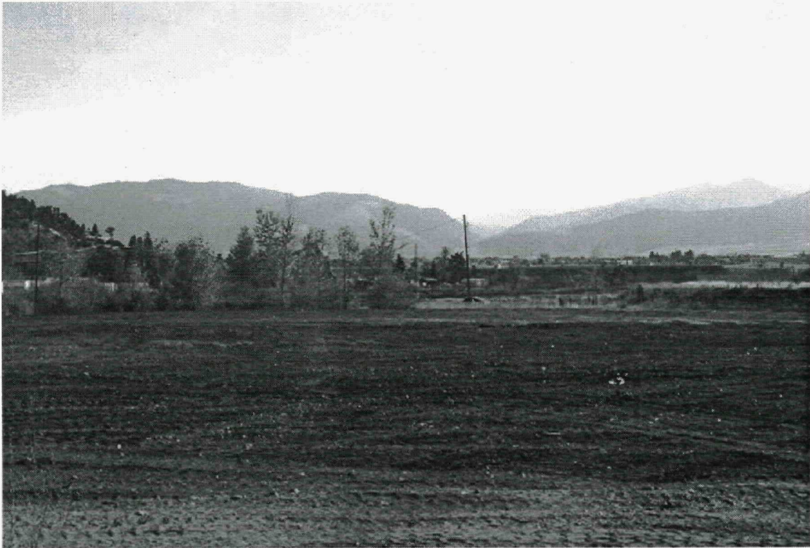
Finished grade of area North of LTU and East of PP-Injection gallery.
