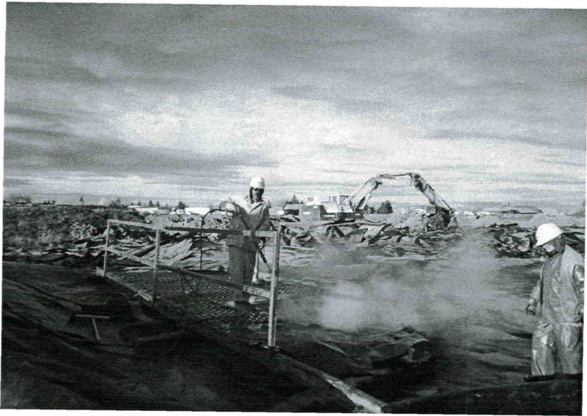
Pressure washing liner stockpiled in the background.
