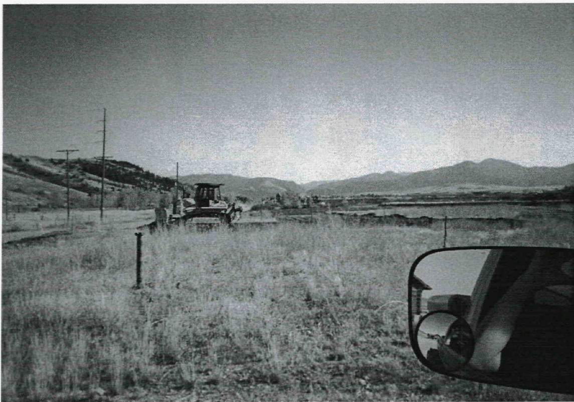
Remaining clean soil placed in low area North of PP-Injection gallery.
