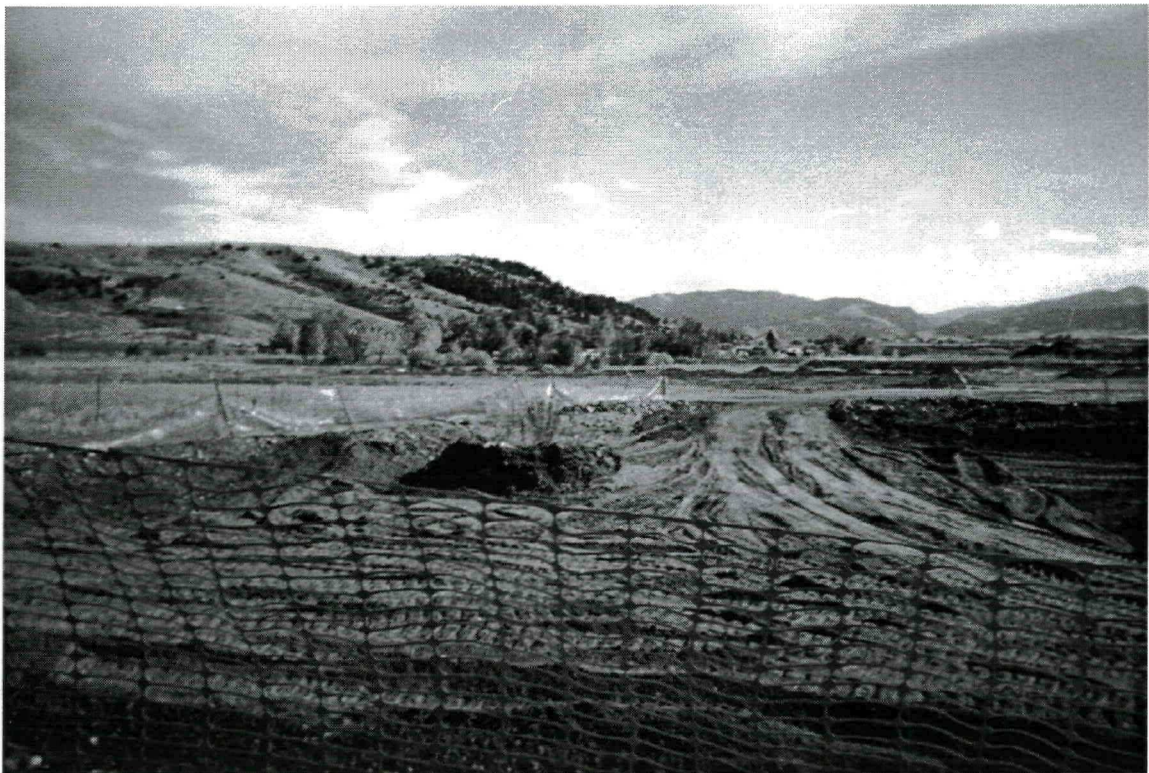
Haul route for relocation of Treated LTU soils into excavated Pit areas.
