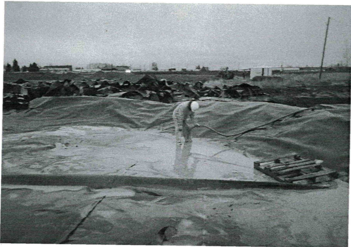
Removal of decontamination water from liner washing area.
