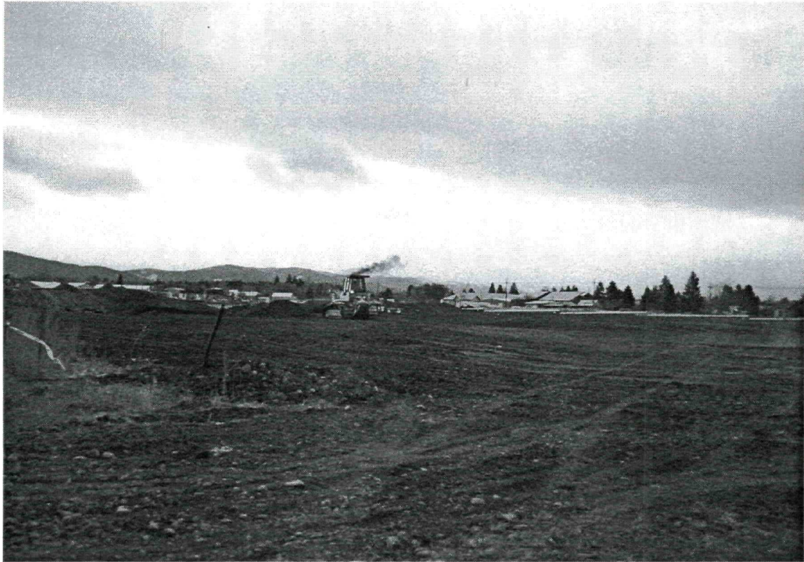
Dozer grading clean soil cover above treated LTU soils.
