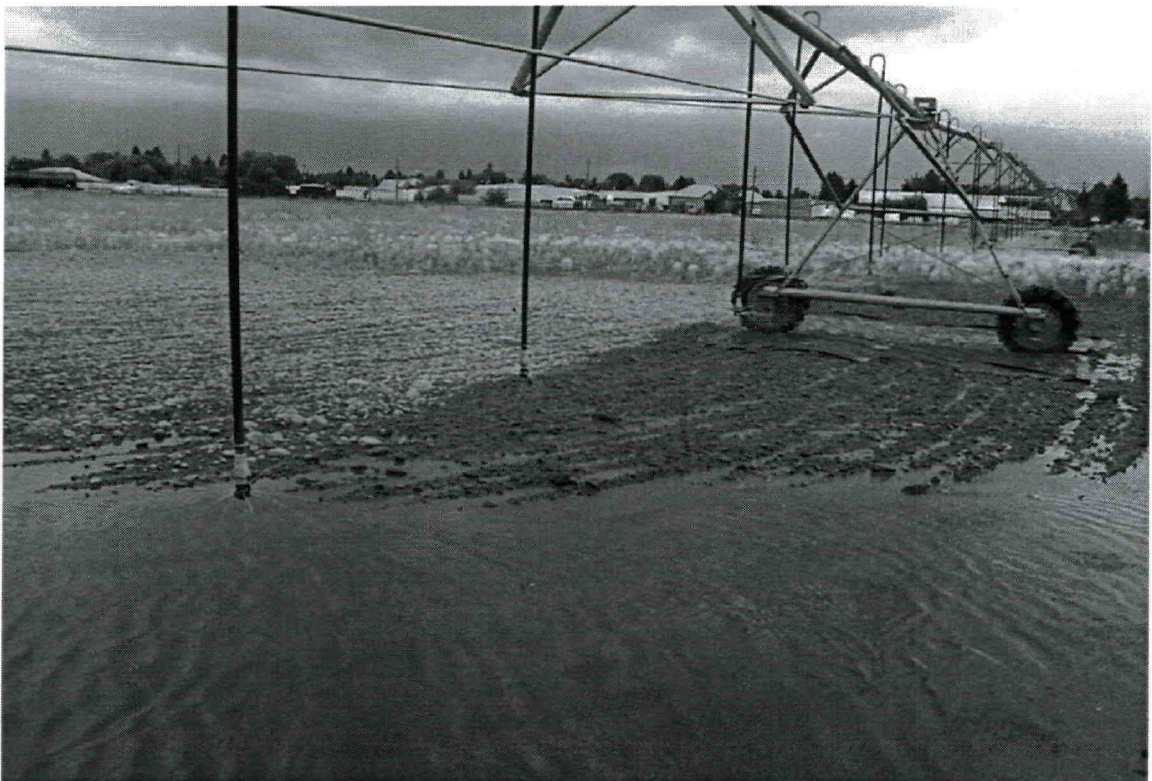
Flushing entire pivot system inside LTU prior to dismantle and removal.
