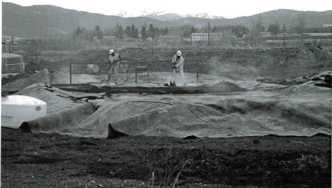
Second liner washing area upon removal of Retention Pond.
