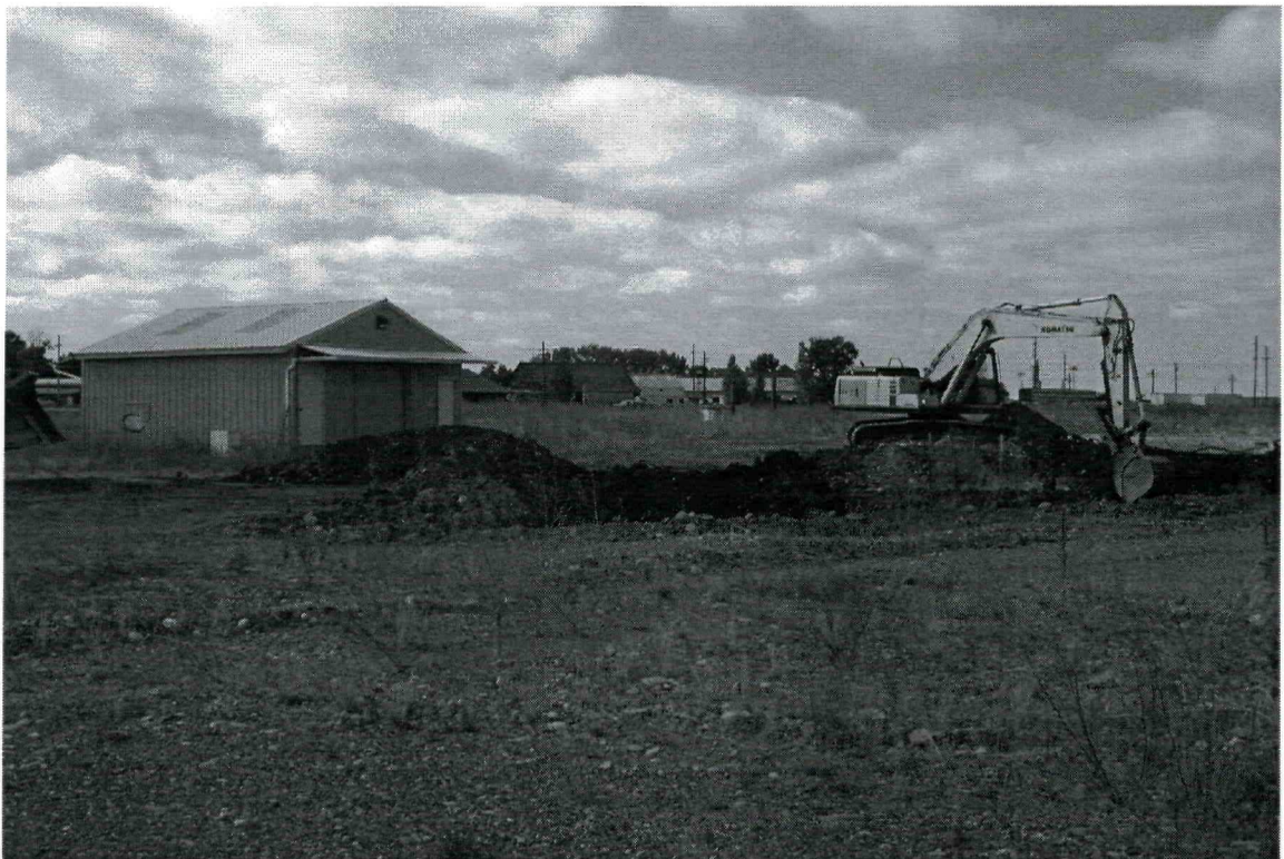
Begin excavation of Pit areas North of Peeler building.
