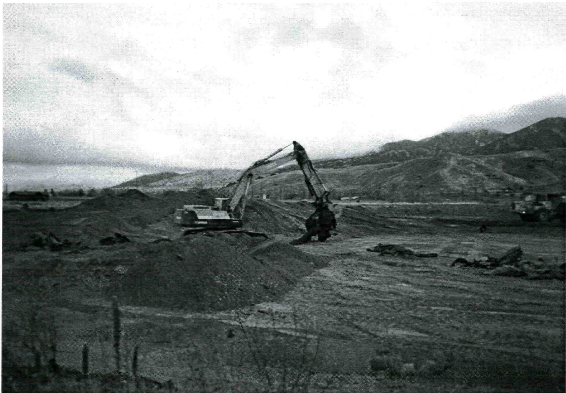
Removing geo-textile fabric from treated LTU soils in LTU.
