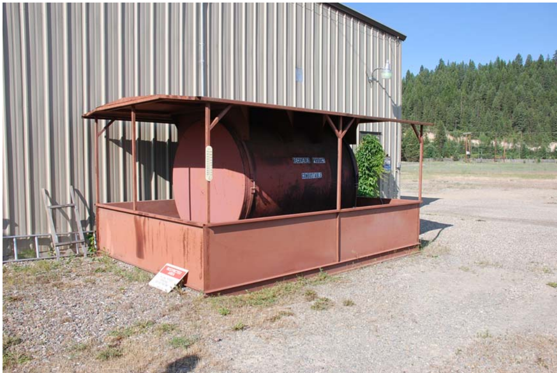
Photo 2: Looking northwest at Source Area Extraction and Treatment System building and recovered product tank.
