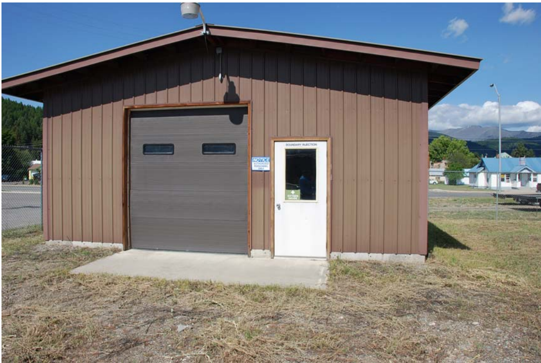
Photo 14: Looking west at Boundary Injection System building.
