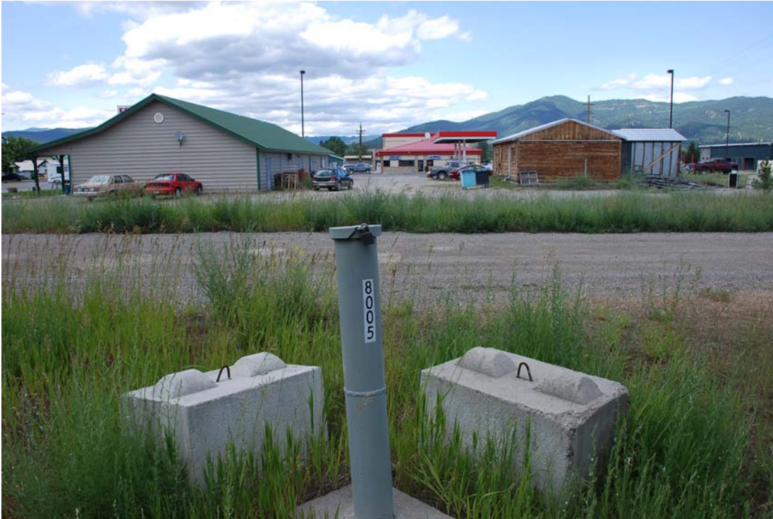
Photo 19: Onsite monitoring well 8005, showing protective bollards.
