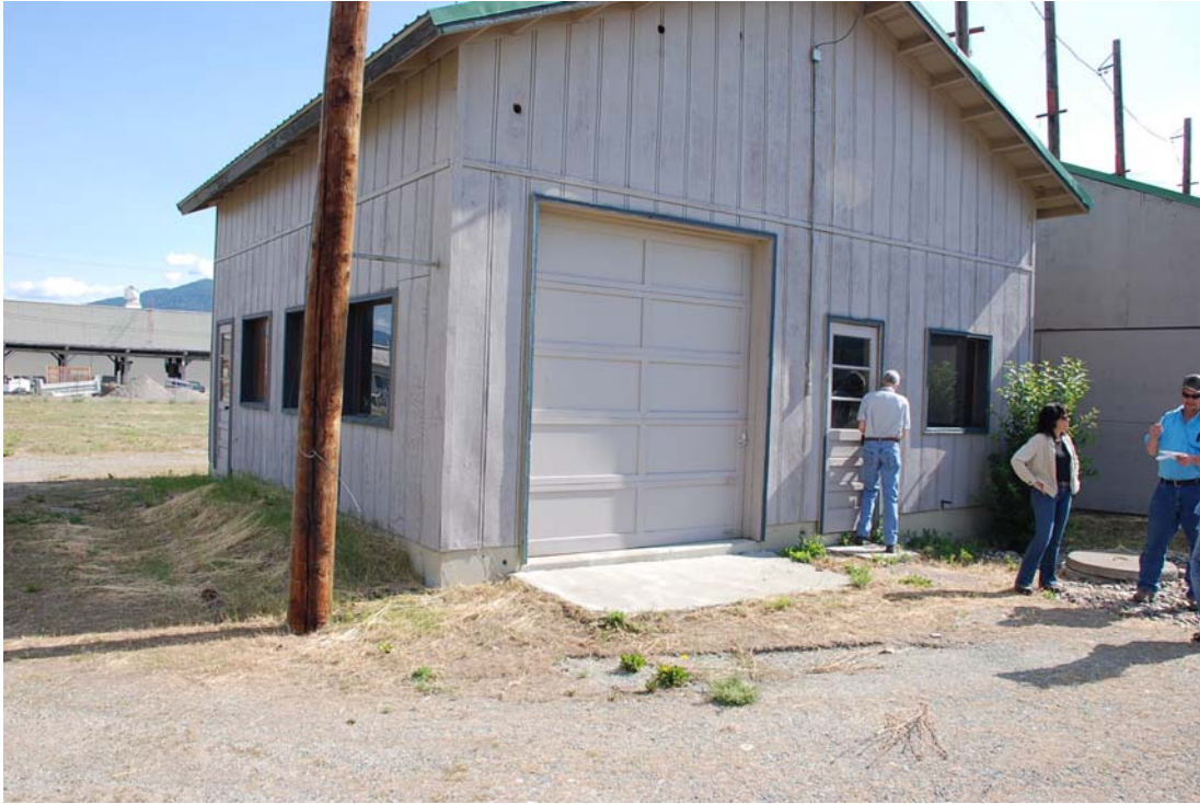
Photo 9: Looking northeast at Intermediate Injection System building.
