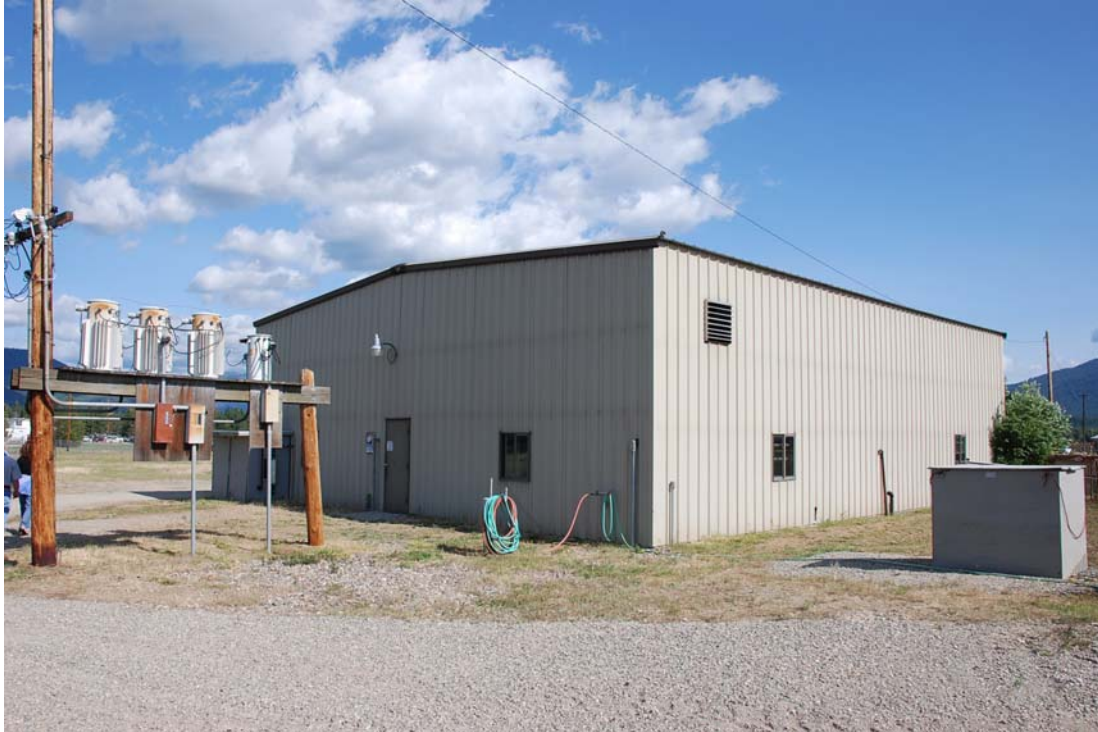
Photo 1: Looking southeast at Source Area Extraction and Treatment System Building.
