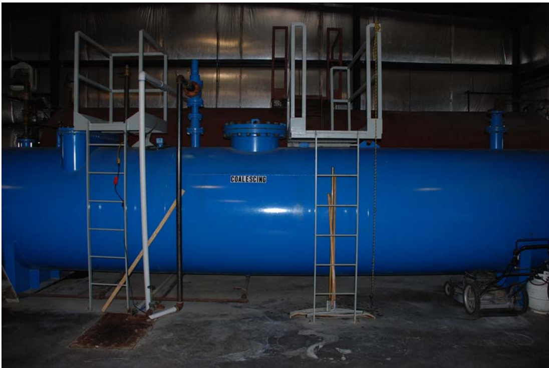
Photo 4: Inside Source Area Extraction and Treatment System building.
