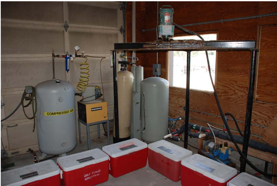
Photo 10: System components inside the Intermediate Injection System building.
