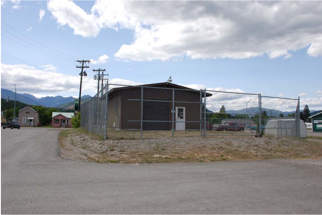
Photo 13: Looking west at Boundary Injection System building.
