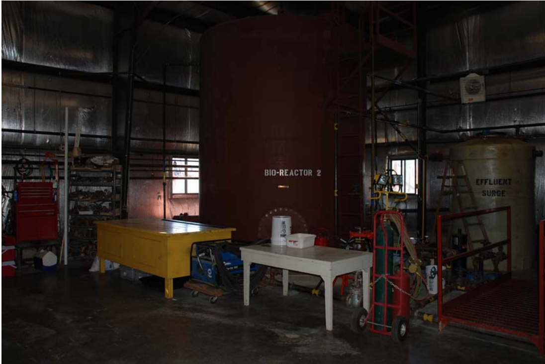
Photo 3: Inside Source Area Extraction and Treatment System building.
