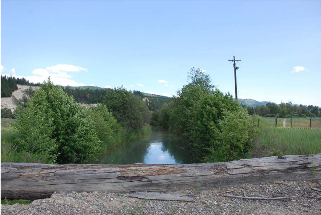
Photo 21: Looking southwest at the Libby Creek Diversion Canal.
