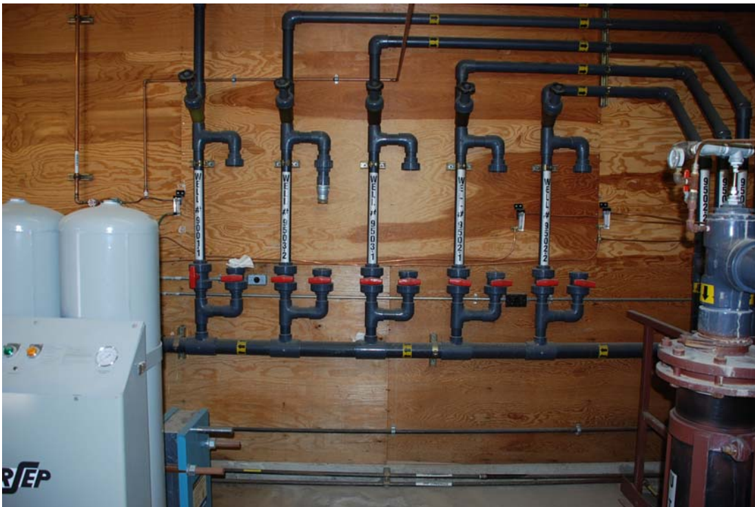
Photo 16: Components of Boundary Injection System.
