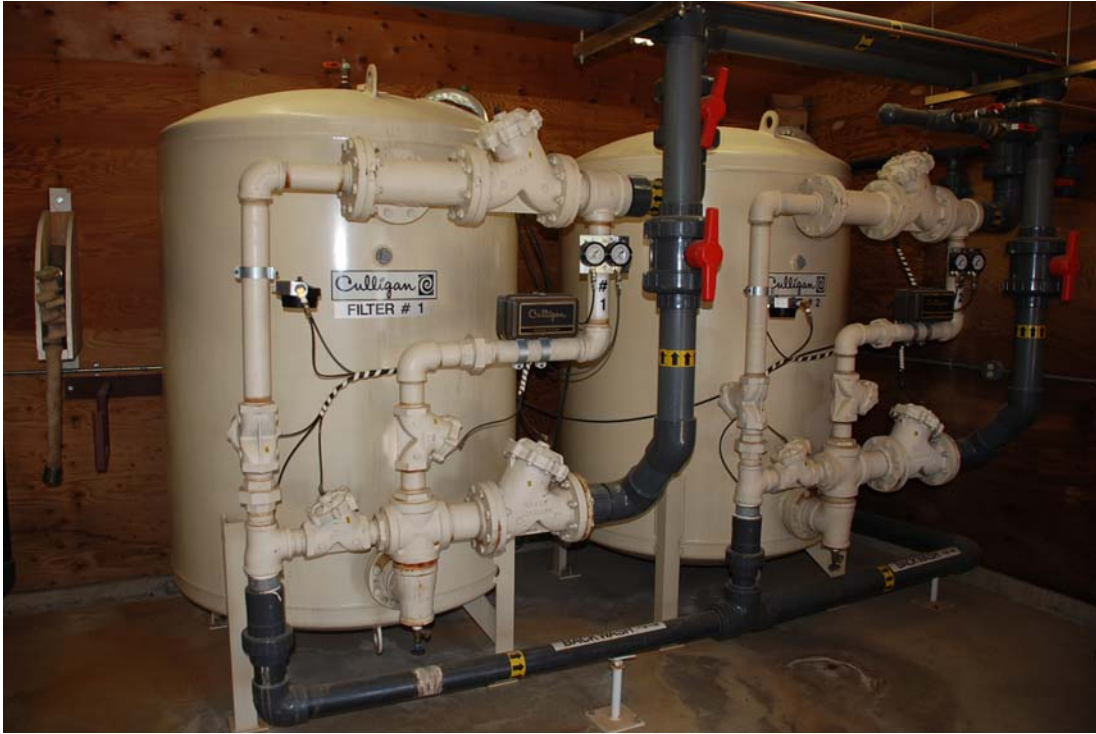
Photo 15: Components of Boundary Injection System.
