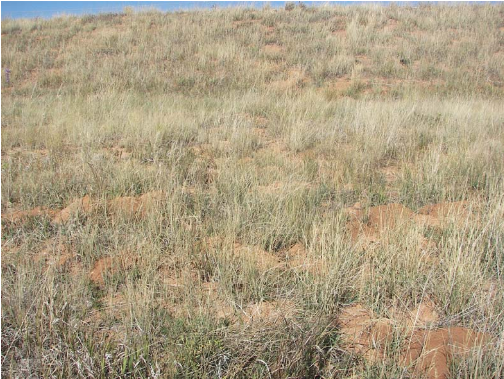
6. Animal burrows on and below the Pond 4 berm.
