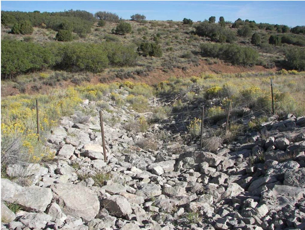
3. Rock-lined drainage between the West Drain Ditch and North Draw.
