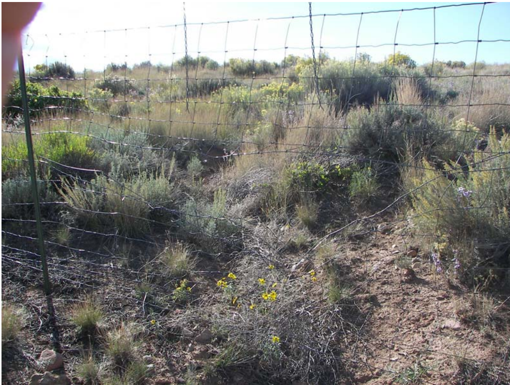
9. Hole in northeast section of wildlife fence.
