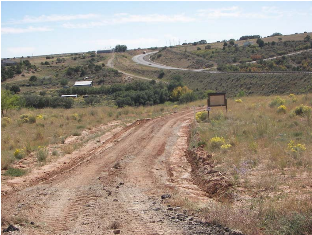
18. Recently graded bike path at former mill site.
