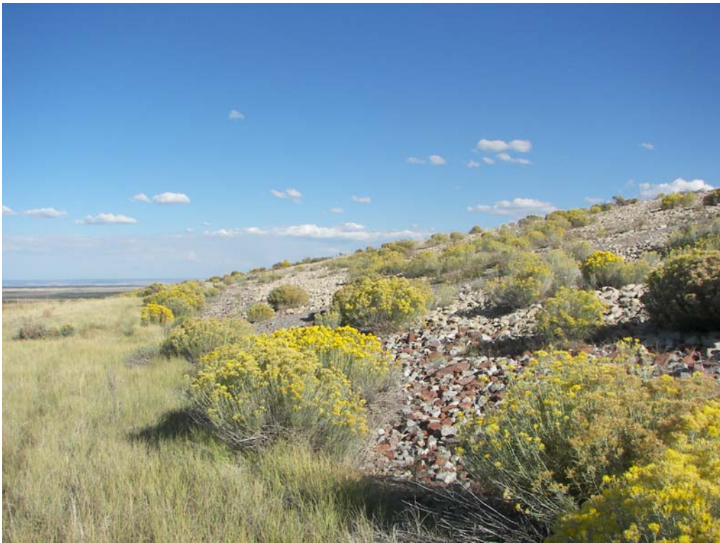
12. Vegetation on rock side slope of repository.
