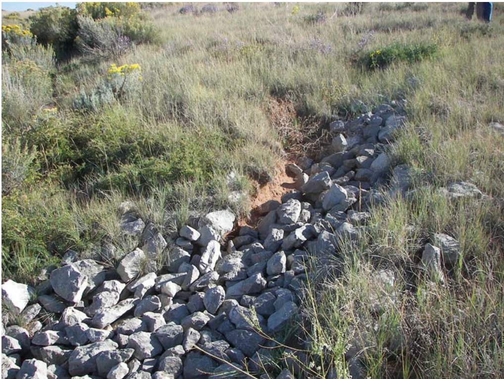
4. Stabilized erosion area near the West Drain Ditch.
