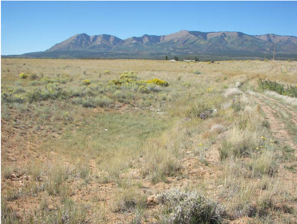
20. Runoff/drainage control structure, Deer Draw Dam.
