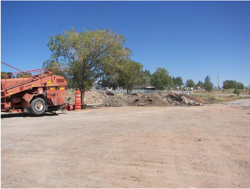
19. Fill materials at City-Owned Property MP-00211.
