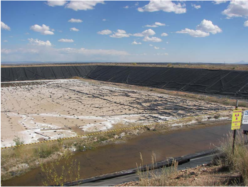
7. Pond 4 showing siltation, vegetation, and standing water.
