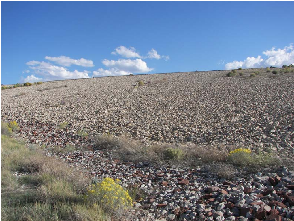
14. Rock side slope of repository and North Toe Trench.
