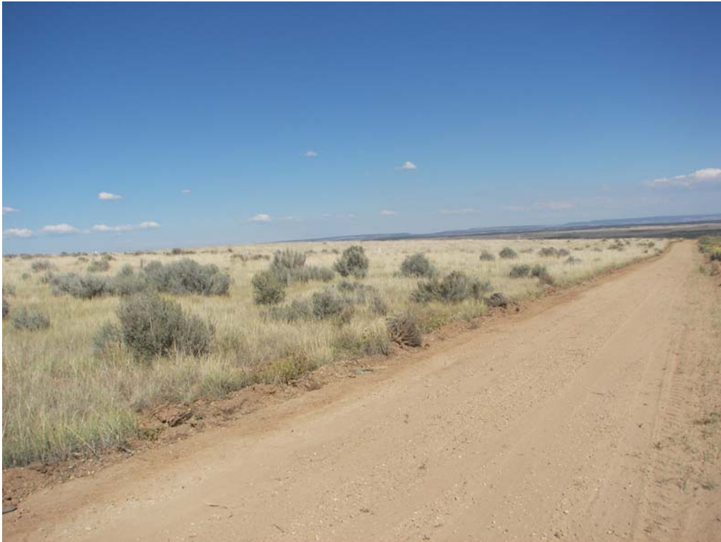
8. Repository cover and recently graded perimeter road.
