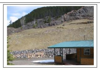
Figure 4. Before and after photographs of the 2004 residential soil removal action showing the stabilized waste rock dump and the reclaimed residential yard at the north end of town.
