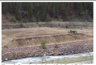
Figure 3. Capped and reinforced Belt Creek Tailings
