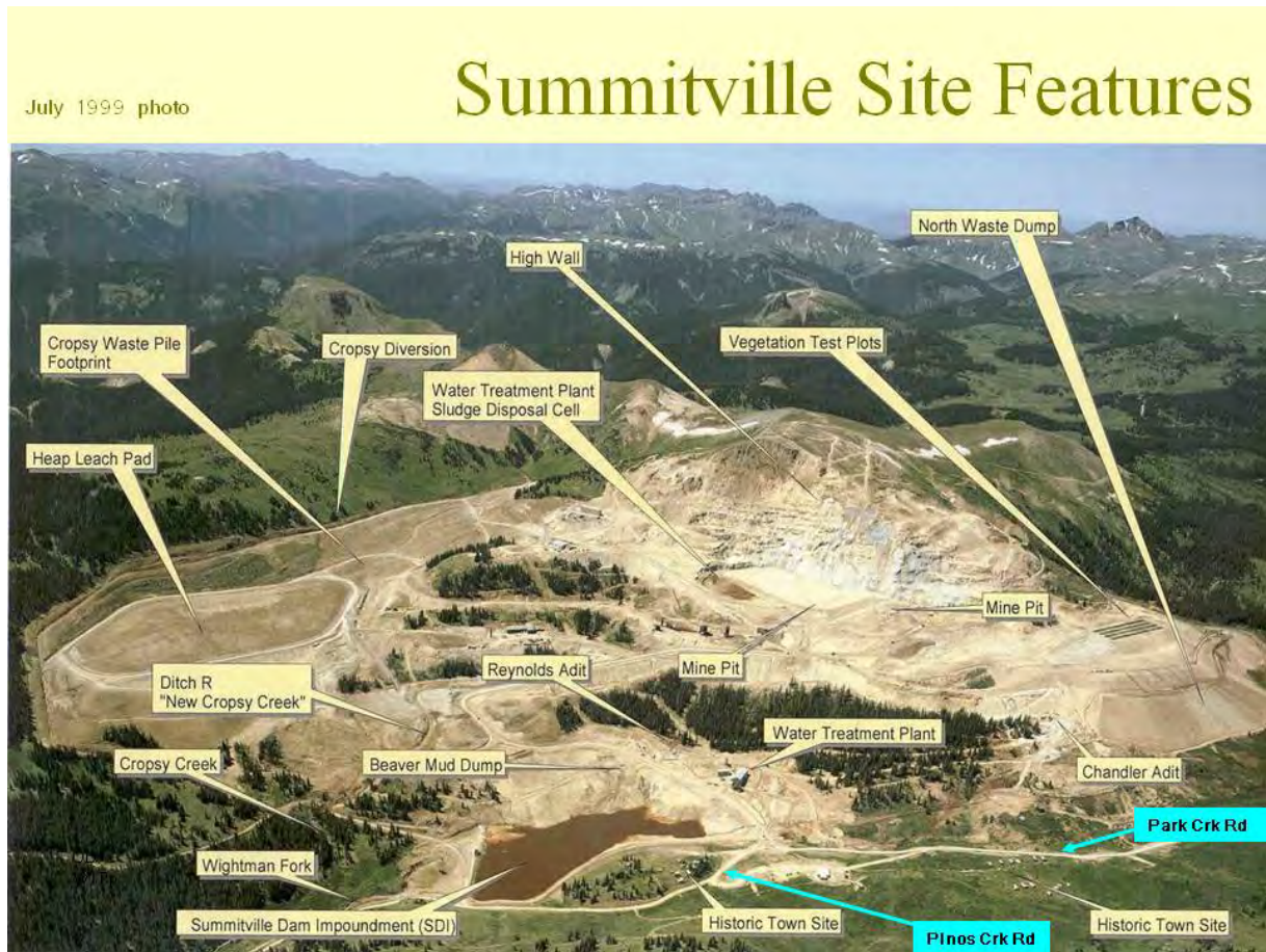
Figure 2: Summitville Mine Superfund Site with HLP (left center), SDI (bottom center), Mine Pits (center), NWD (right center), and interim WTP (right of SDI) during 1999.
