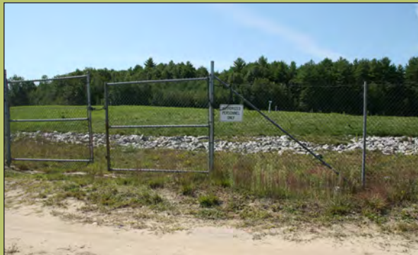
PICTURED: A fenced portion of the site, along with a cautionary sign limiting access to the site. (source: EPA)
