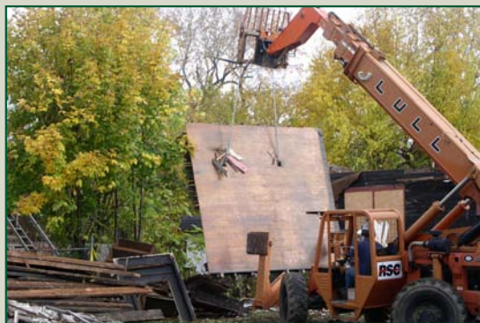
City of Cleveland deconstructing an abandoned building as part of its Deconstruction Initiative program.
