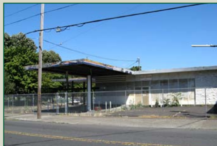
The June Key Delta House site before redevelopment construction begins.
