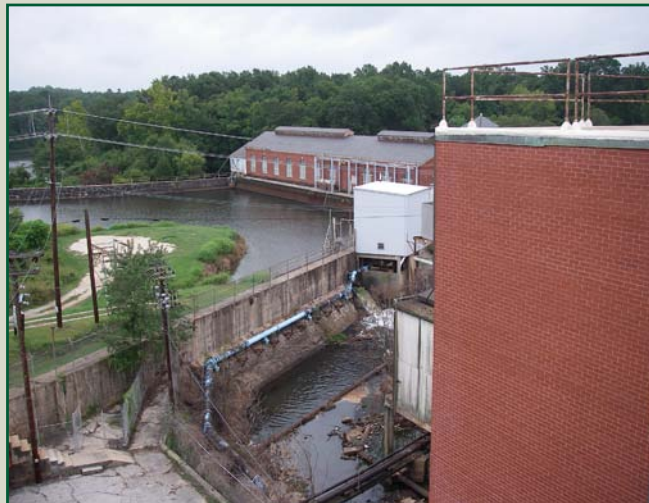
A view of Langdale Mill.
