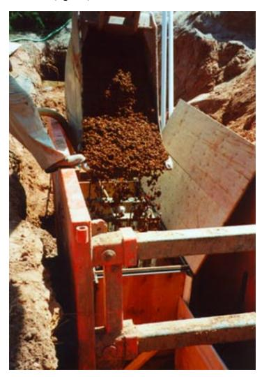
**Figure 5.2.** Placement of AFO barrier material into the gate structure of the permeable reactive barrier, Fry Canyon, Utah.
