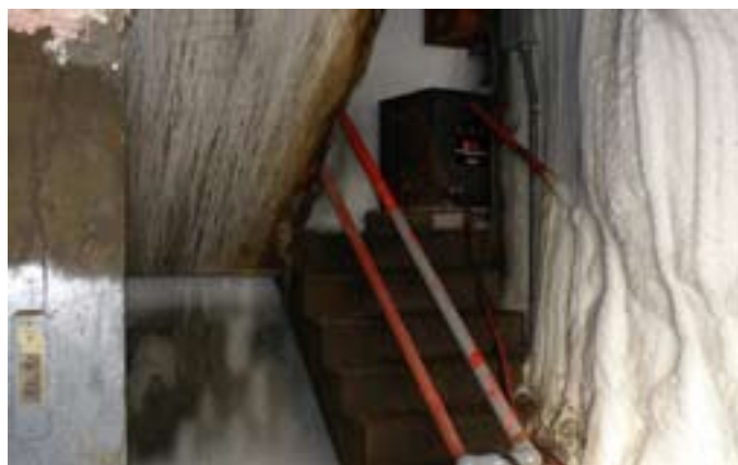
Ice Buildup Blocking Stairway
