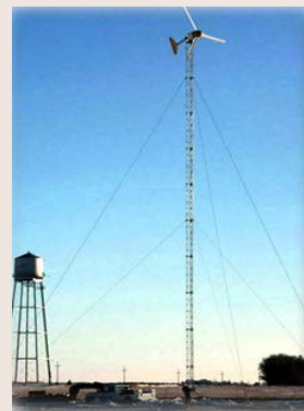
A 10 kW wind turbine powers a ground water circulation well
