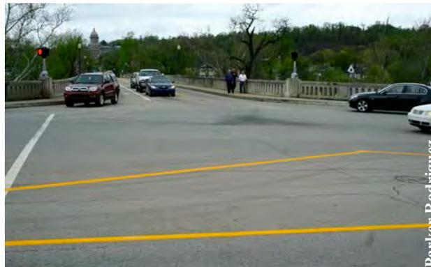
**Figure 22:** The painted median on Main Street offers little protection to pedestrians trying to cross the 60-foot-long crosswalk.
