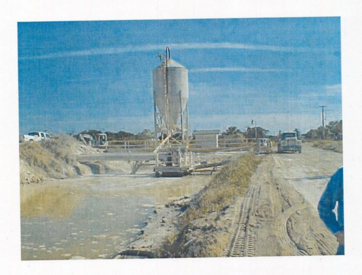
Initial liming station at a ditch connecting pond 6 and pond 1.
