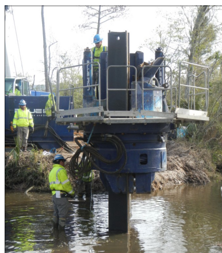
Sheet piling, using interlocking metal plates, are installed in Turkey Creek for bank stabilization.
