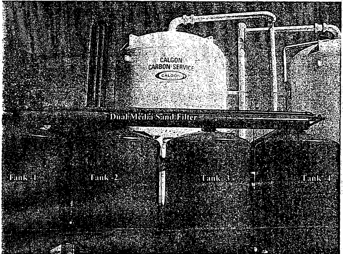
Photo 8 - Sand and Carbon Absorption Filters
