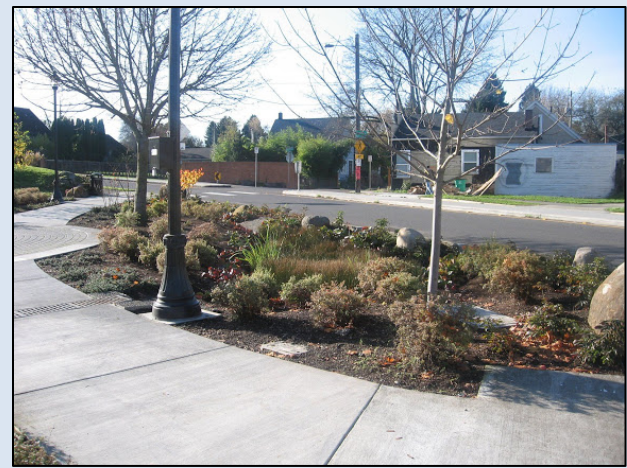
Exhibit 3-1: An Infiltration Basin in an Existing Neighborhood. This bioswale and infiltration basin includes plantings and trees that help collect and treat stormwater runoff that flows off the sidewalks and streets in this neighborhood.
