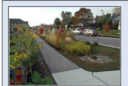
Exhibit 3-5: A Swale Integrated into a Roadway. Some of the streets in the Green Zone, such as Wadsworth Avenue, could accommodate a roadway swale like the one pictured above. The swale would help capture and treat stormwater and also be aesthetically pleasing.
