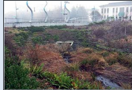
Exhibit 3-3: A Block-Scale Rain Garden. Reusing vacant blocks as rain gardens can help cities capture stormwater on site and reduce the amount of stormwater that enters the city's sewer system.
