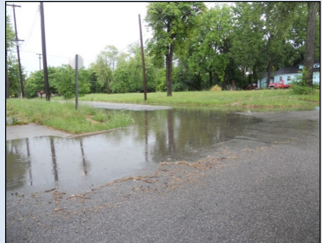
Exhibit 3-2: Stormwater Ponding in the Green Zone. By using green infrastructure, which collects stormwater and helps filter it back into the ground, Saginaw can reduce the amount of water that collects on city streets.
