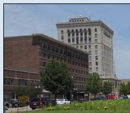
Exhibit 1-1: Recent Redevelopment in Downtown Saginaw. The Savoy Bar & Grill (top) and the conversion of the Bancroft Eddy Building (bottom) into 150 units of luxury housing units are examples of recent redevelopment in downtown Saginaw.
