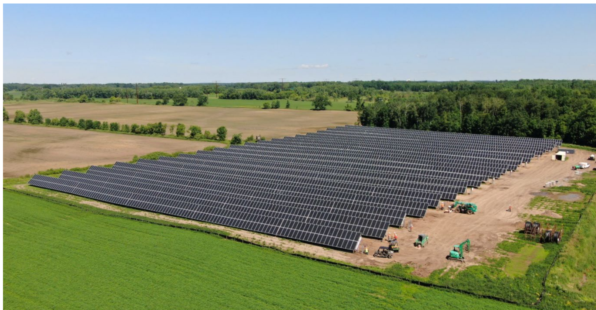
The new 1.852 MW solar field at Green Valley Dairy was installed by Arch Electric and began operation in September 2020. Photo Credit: Arch Electric
