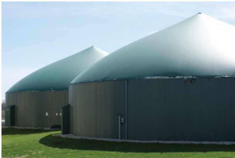
Above-ground complete mix digesters at Green Valley Dairy. Photo Credit: Energy Center of Wisconsin
