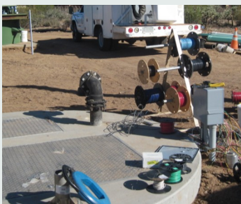
Sells Lift Station Construction Project
