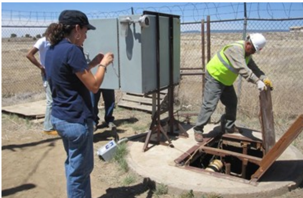
Ramah Lift Station Inspection, Navajo Nation May 2011.
