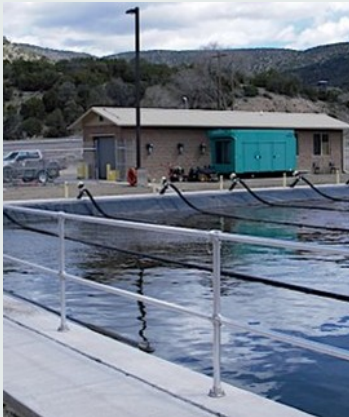
Nambe Pueblo Wastewater Treatment System Construction Project
