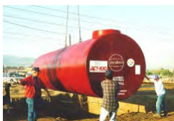
Underground storage tank
