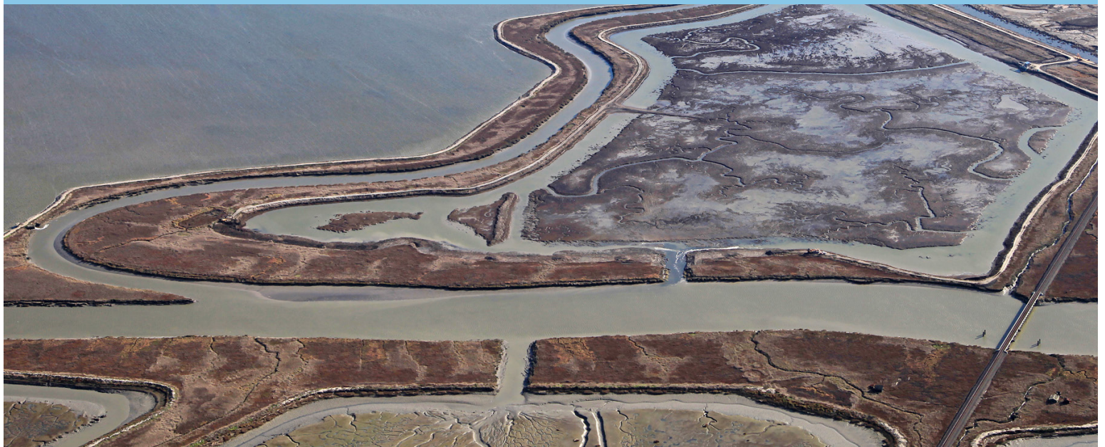
Restoration of South Bay Salt Pond A 17 near completion. Photo: McMillen Ltd.
