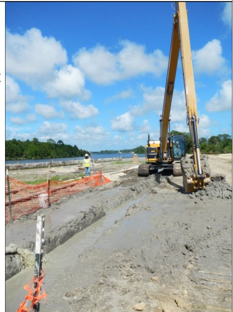
Earth-moving equipment constructs special trench and wall to reduce pollution entering Turkey Creek.
