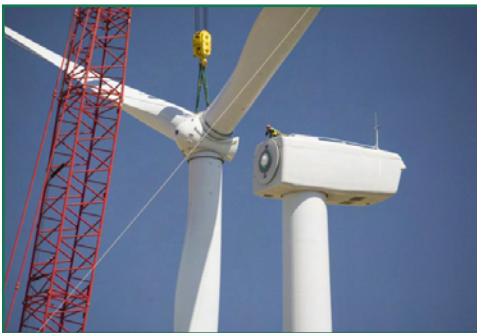
A 1.5 MW wind turbine being installed
