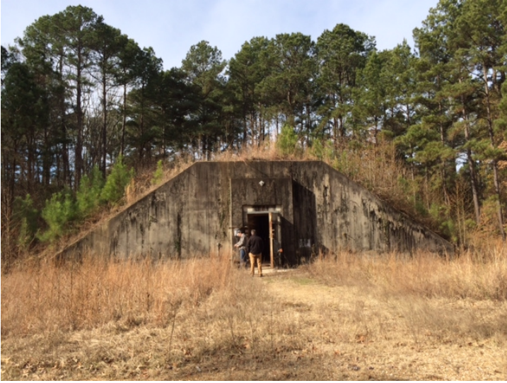
Photo 4: Example of explosive storage magazine at Camp Minden
