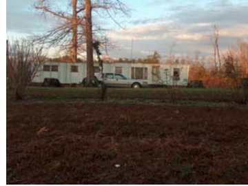
Figure 2. Dilapidated Trailer in King William County
