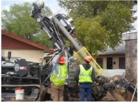
Figure 6. Sheet pile Electrode Installation
