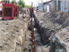
Figure 7. Horizontal Electrode Installation
