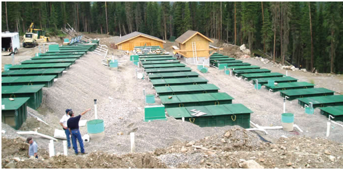
Advanced treatment units
