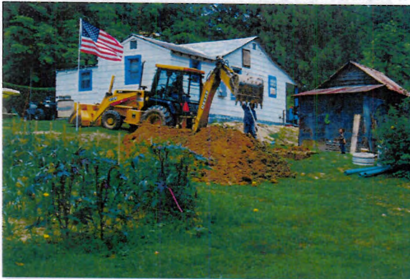
Beginning installation at home on Flat Creek
