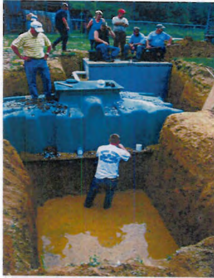
Peat module installation
