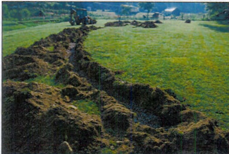
Preparation for low pressure pipe system
