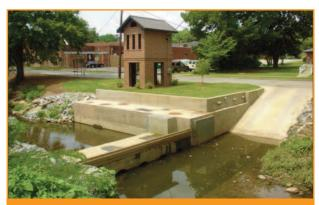
WWETCO Compressed Media Filter and Flow Controls with ultraviolet disinfection for Weracoba Creek stormwater treatment in Columbus, Georgia
