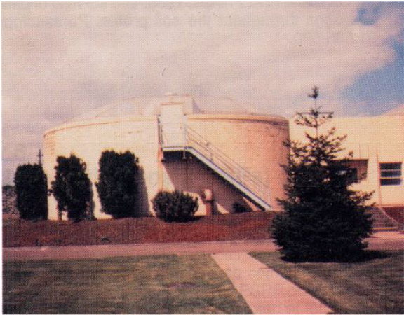
Digester in Vancouver, Washington.
