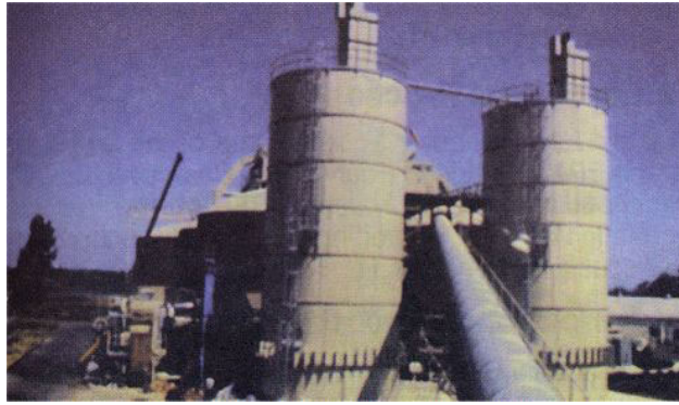
Taulman Weiss in-vessel composting facility in Portland, Oregon.
