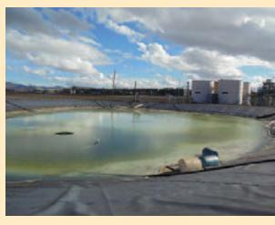
A lined pond at the Tronox facility in Henderson, Nev., still contains residual perchlorate from the pond's former use in the manufacturing process.
