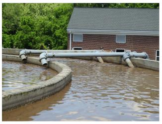
surface in the first ditch. Results were immediate, decreasing DO by as much as 1.0 mg/L where the influent and RAS enter the ditch.
