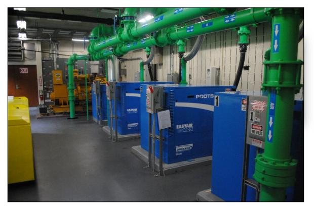
With the risk of mechanical equipment failure reduced, the upgrade made it possible to deviate from conventional aeration methods and experiment with cyclical aeration. The blowers could now be controlled based on DO levels and/or timers. ORP readings are used to monitor performance of the cyclic aeration system.
