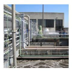
Upgrade was through operational changes only. Aeration was decreased in initial zones (1 and 2 of 6) in each of the three operating nitrification tanks to create an initial low-DO region for simultaneous nitrification and denitrification. DO concentrations were decreased from 2.5 mg/L to less than 0.5 mg/L, average.
