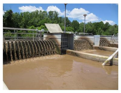
experiment with operating the ditch aerators in an on/off operation mode. A 24-hour timer with 15 minute on/off cycles was used in initial tests to determine the effectiveness of this approach in maintaining the DO at the desired levels. The timer was wired to one of the two available aeration motors. The timer cycled on/off effectively, but lacked the ability to alter the speed of the motor. Plant performance improvements were marginal with this modification.
