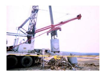
Figure C-10. LFG Well Drilling.
