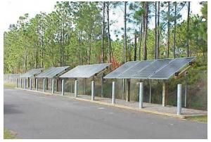
Figure C-2. Photovoltaic Solar Panel Installation.
