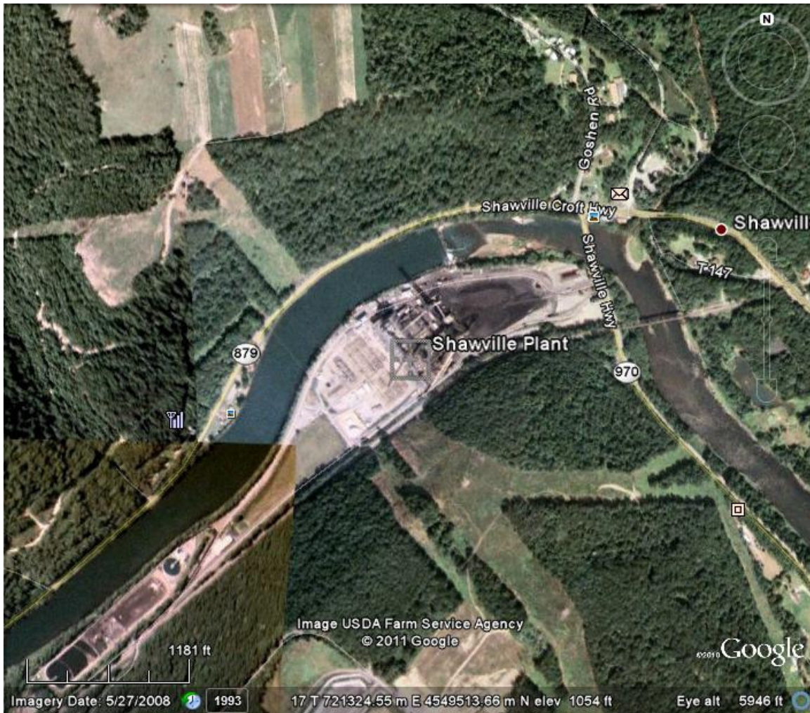
Figure 1. GenOn Shawville Coal Plant
