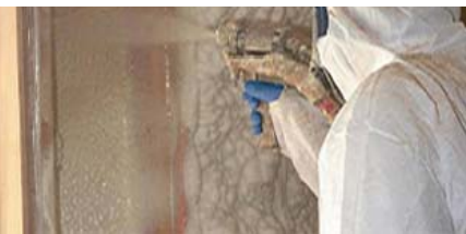
SPF spray application on wall
