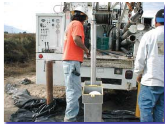
Drilling groundwater monitoring well.
