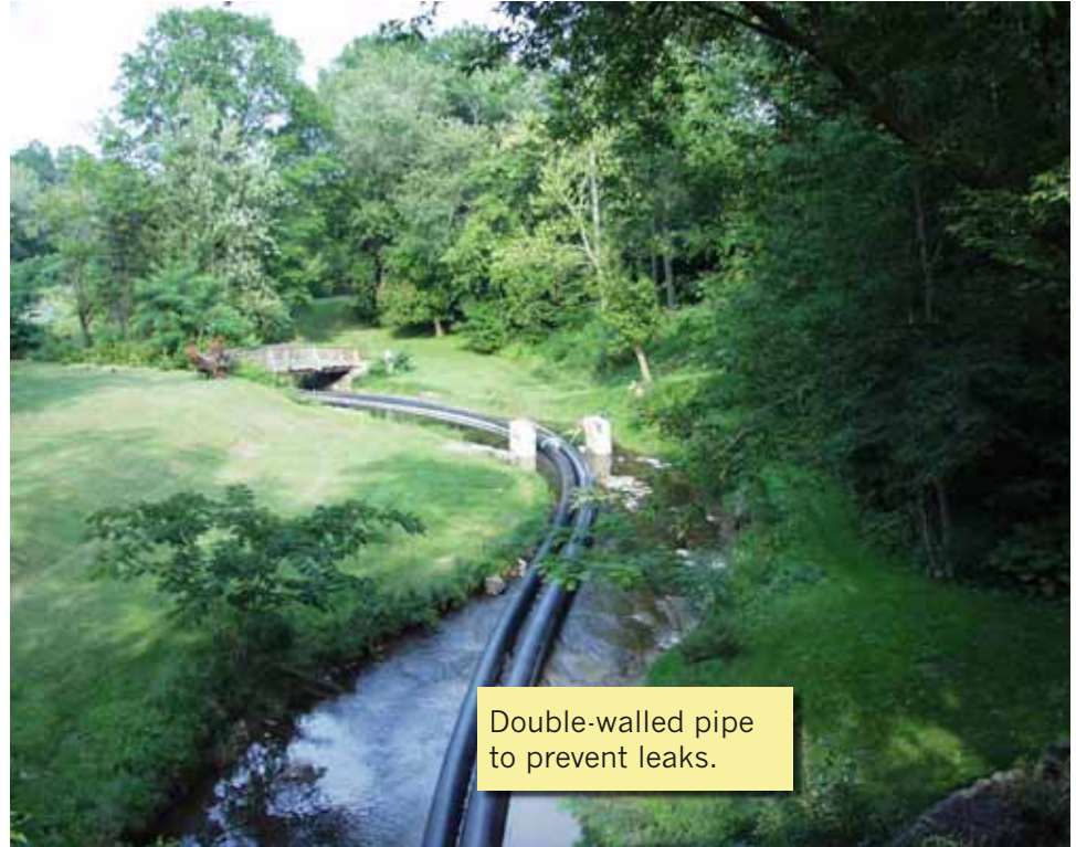
Pipeline to the landfill.
