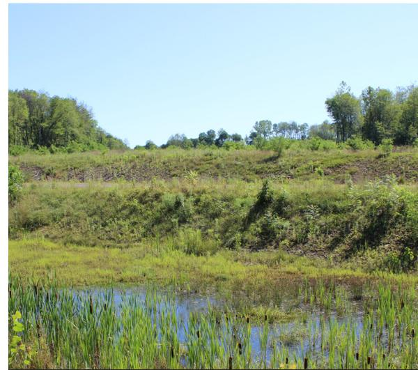
Earth Conservancy oversaw construction of this stormwater basin to manage acid mine drainage at the Hanover 9 site.
