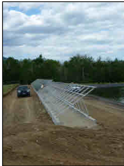
FIGURE 3. RED LODGE SOLAR ARRAY UNDER CONSTRUCTION
