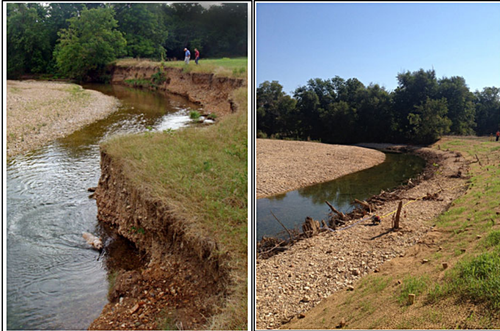
FIGURES 6 AND 7. BEFORE AND AFTER PHOTOS OF REPAIRED SITE ON ILLINOIS RIVER
