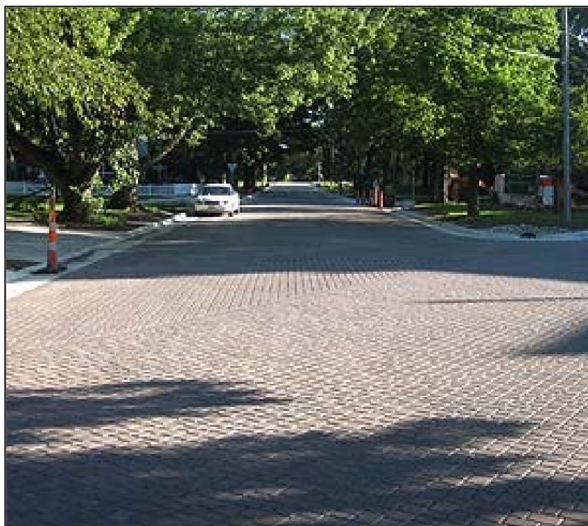
FIGURE 1. CHARLES CITY GREEN PERMEABLE PAVING PROJECT
