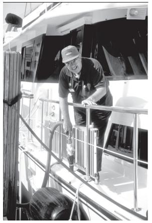
Figure 4-20. Pumpout system at Hall of Fame Marina (Florida). Accommodating dozens of yachts more than 100 feet LOA, the marina's pumpout system includes below-dock sewer pipes and connectors of each slip (USEPA, 1996: *Clean Marinas—Clear Value*).
