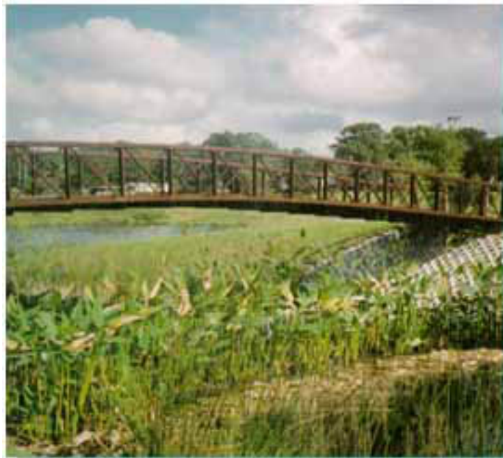
Constructed wetlands are being effectively used to help protect the quality of urban lakes by improving the quality of stormwater runoff in urban areas such as at the Greenwood Urban Wetland, a former dump site, in Orlando, Florida.
