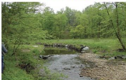
Stream restoration in Prince George's County, MD
