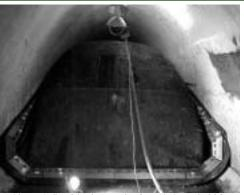
Photo: Inflatable dam at the Sneads Branch CSO Courtesy of LJCMSD
