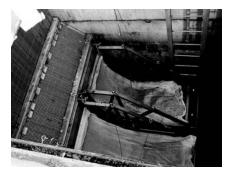
In 1999, North Bergen Municipal Utilities installed numerous mechanical screen bars and netting systems to control solids and floatables in CSOs. The facilities cost \$3.3 million and annually cost \$57,373 to operate and maintain (2002 dollars).
