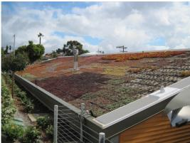
Figure 16. Green Roof with Fully Contained Trays on a Highly Sloped Roof.
