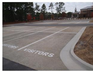
Figure 12. Pervious Concrete Parking Stalls.
