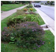
Figure 7. Bioretention Incorporated into a Right-of-Way.
