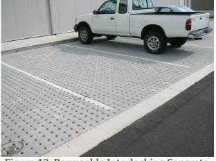
Figure 13. Permeable Interlocking Concrete Paver Parking Stalls.
