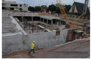
Cast-in-place Concrete Tank Figure 17. Examples of Underground Detention Units.
