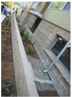
Figure 10. Flow-through Planter Box Attached to Building.
