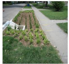
Figure 8. Bioretention Incorporated into Traditional Parking Lot Design.
