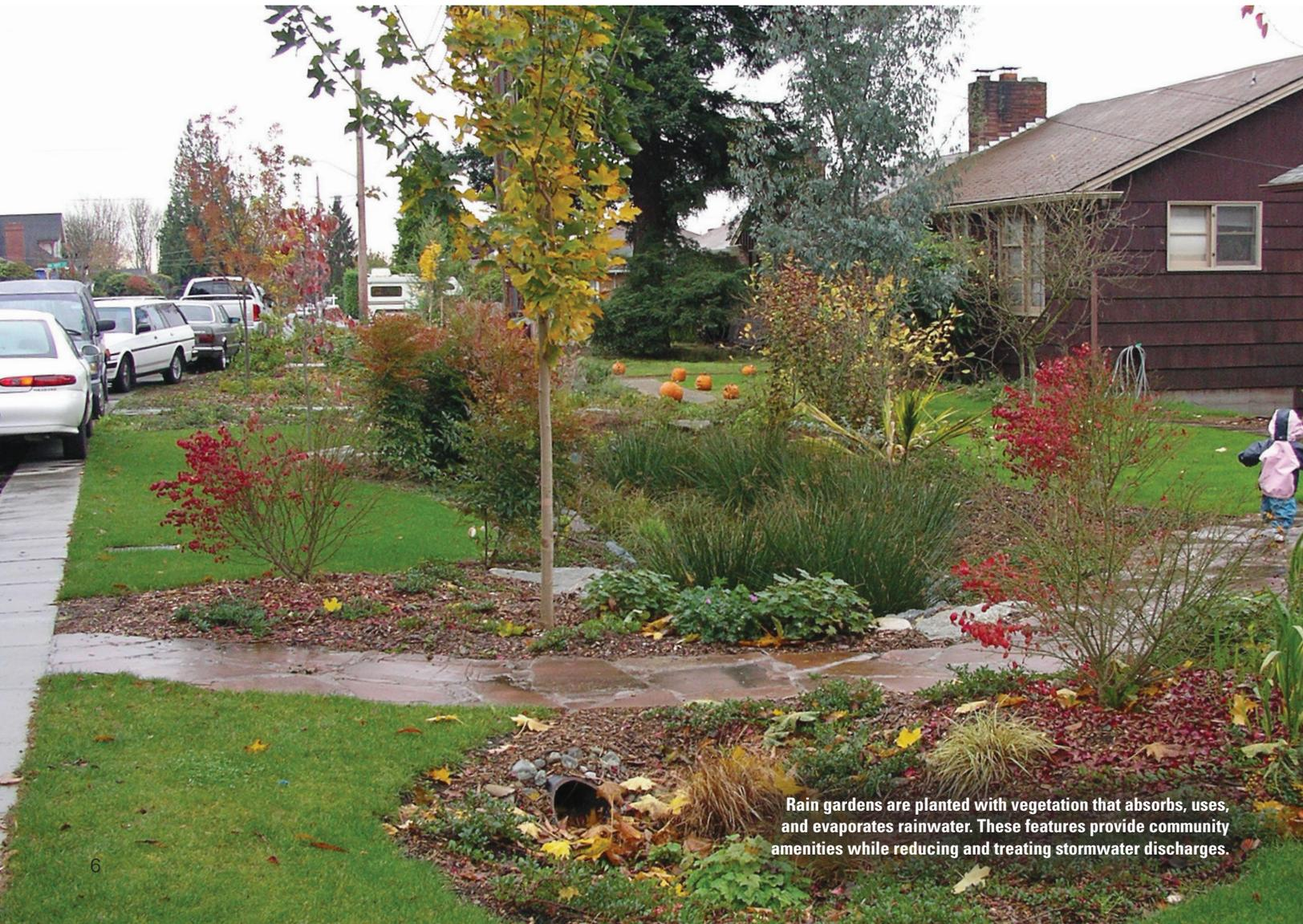
Rain gardens are planted with vegetation that absorbs, uses, and evaporates rainwater. These features provide community amenities while reducing and treating stormwater discharges.
