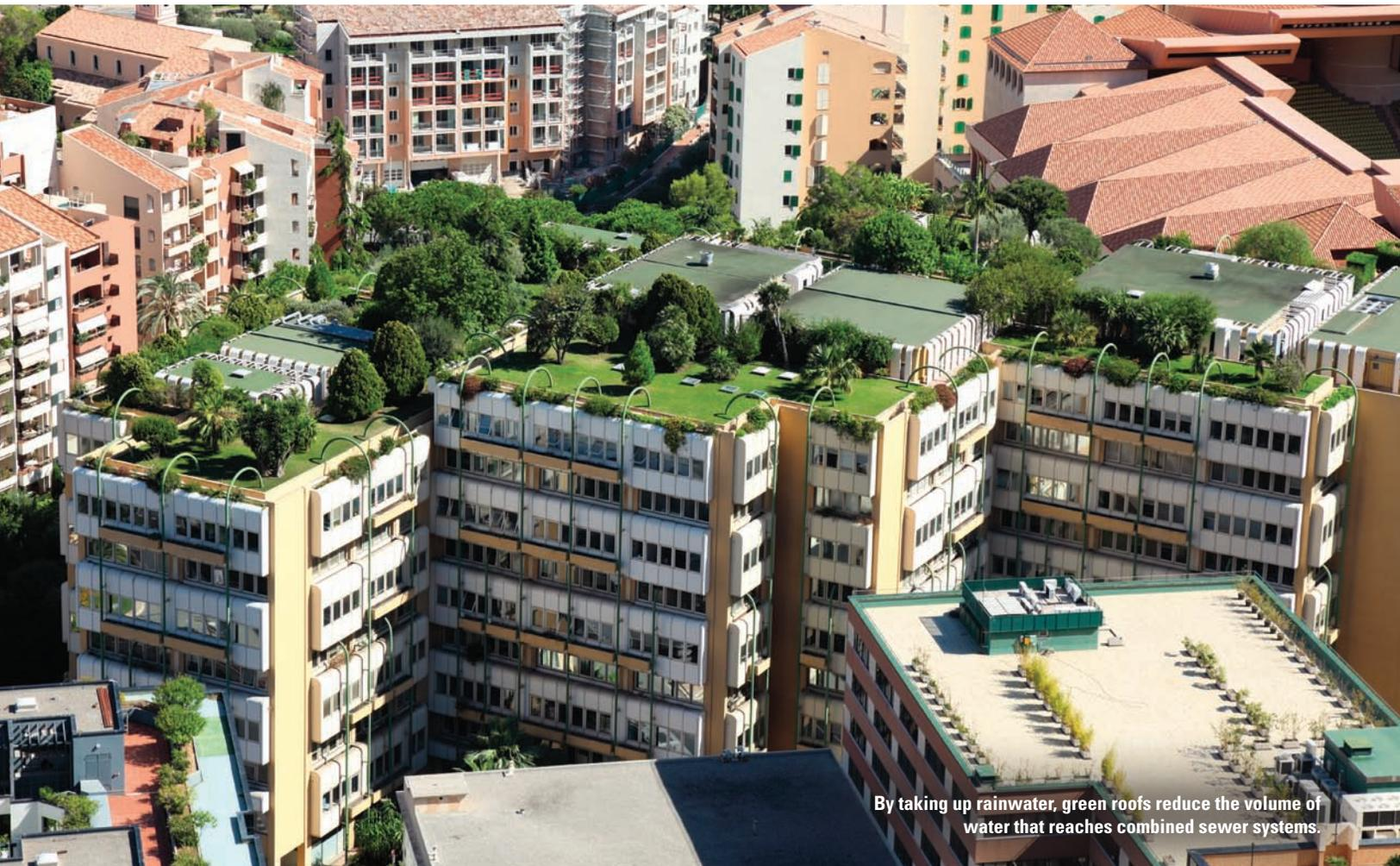
By taking up rainwater, green roofs reduce the volume of water that reaches combined sewer systems.
