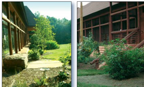
Figure 2. Project partners installed rain gardens along the walls of the Reinhardt College Funk Heritage Center to collect and store roof drainage.
