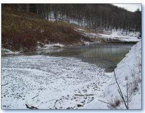
Figure 1. This limestone pond treats AMD in the Miller Run watershed.
