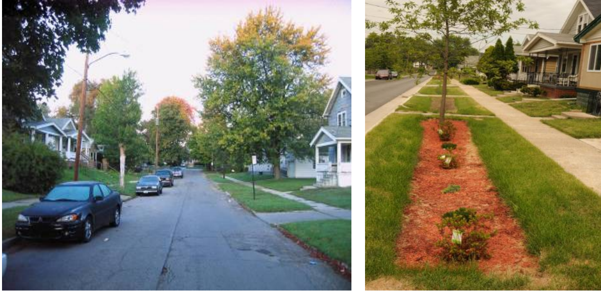
Figure 9. Before and After Bioswales on Maywood Avenue
