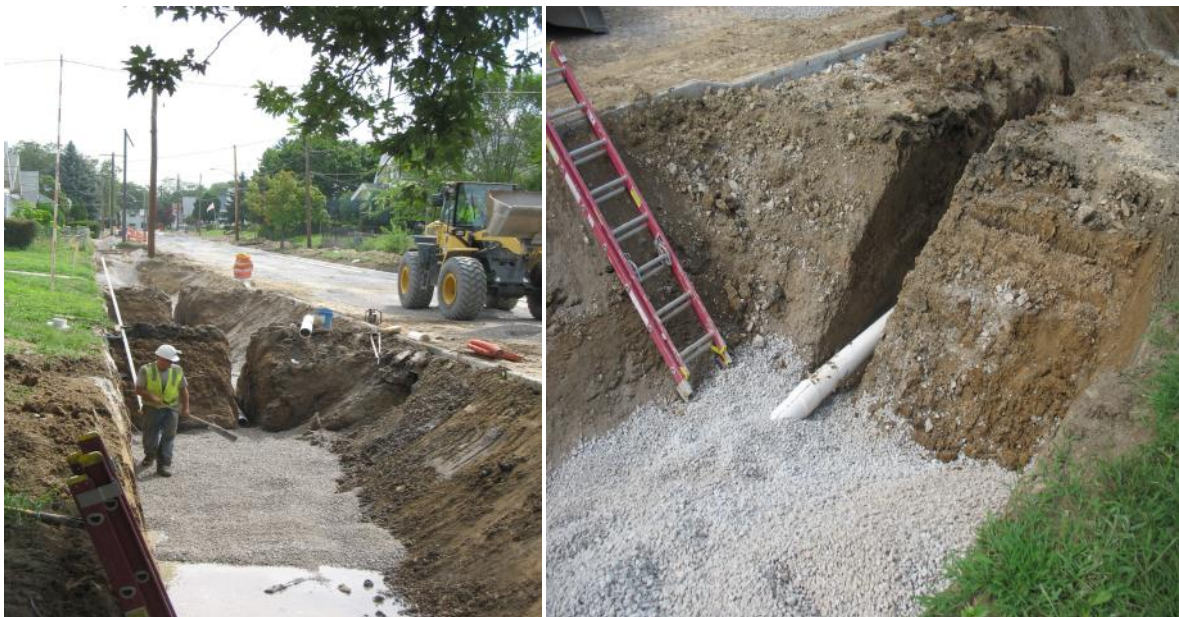
Figure 13. Construction in Clay Soil
